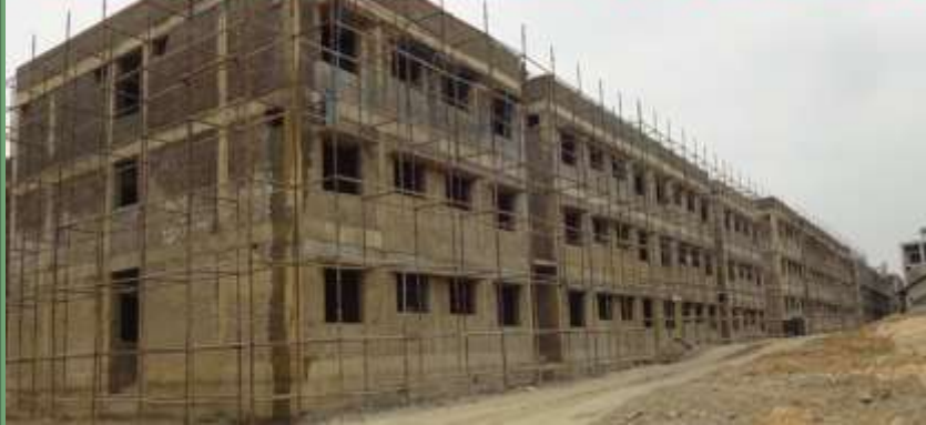
NARIMEDU SCHEME (GROUP-I) IN PUDUKKOTTAI
