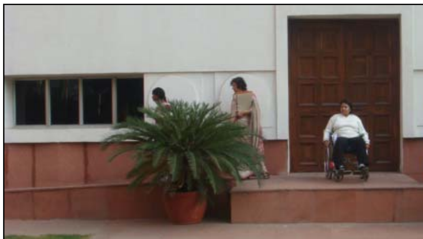
Existing ramp without handrails & guard rail
