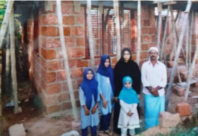
BLC New House construction
