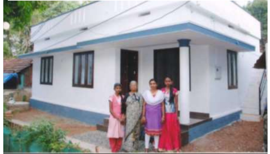
BLC New House construction
