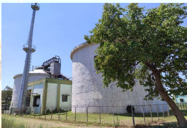
Digester & Equipment Building Of 95 MLD STP at Basarke Bhaini, Khapper Kheri Pind, South - Zone
