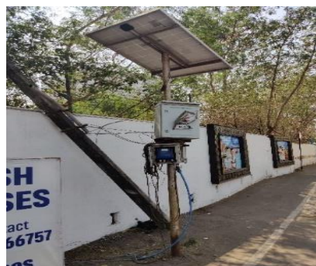
Figure B5: Bulk meters reader and transmitter
