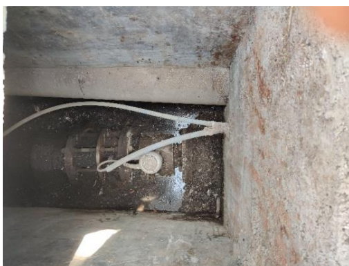
Figure B4: Bulk meters with sensor at entry of DMA
