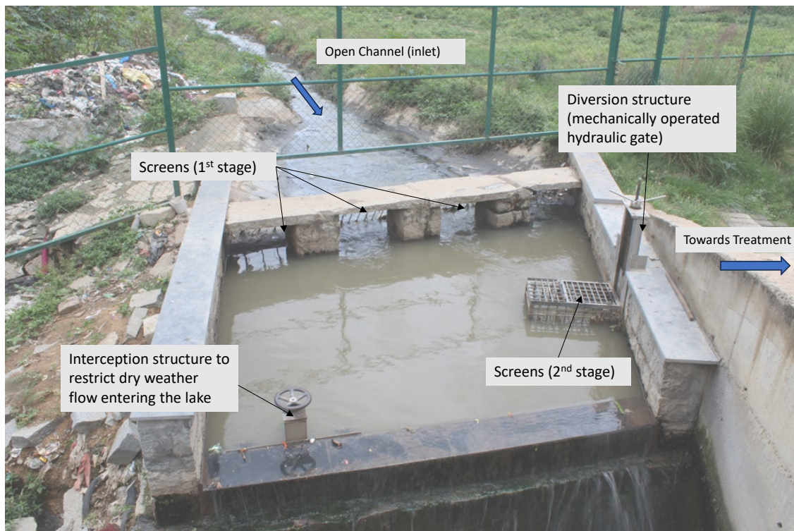
Figure 13. Interception & Diversion structure at Mahadevapura Lake, Bangalore (Source: CDD India)
