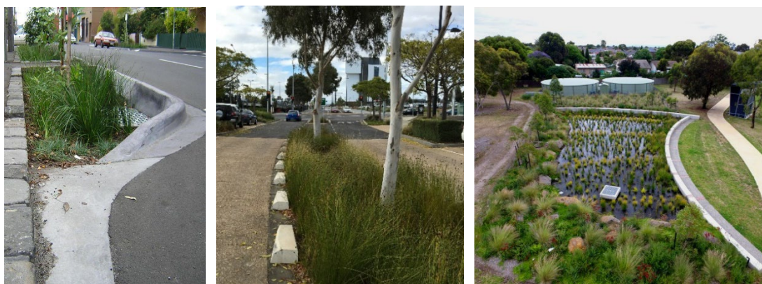
Figure 44. Application of biofiltration technology – Street scale raingarden (left), street scale linear swale (middle) and end-of-pipe biofiltration basin (Source: Spiire)
