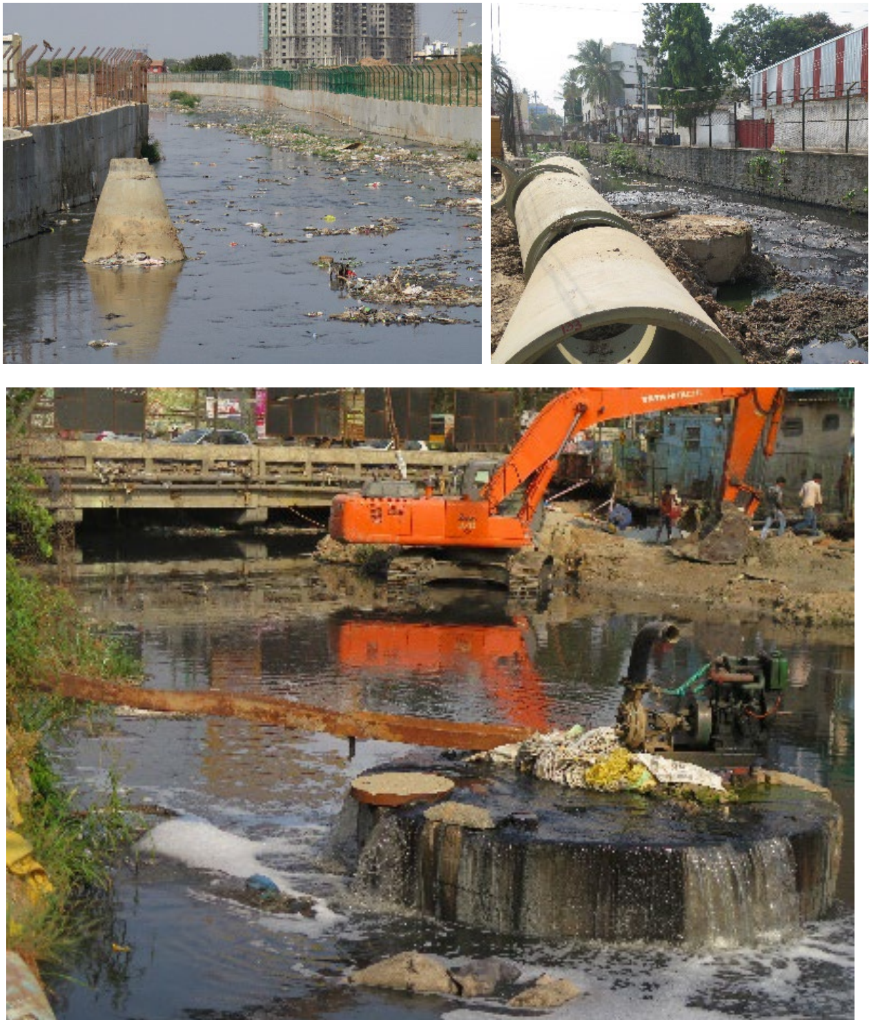
Figure 6: Used water pipelines laid within the stormwater drain and prevalent solid waste dumping in drains
