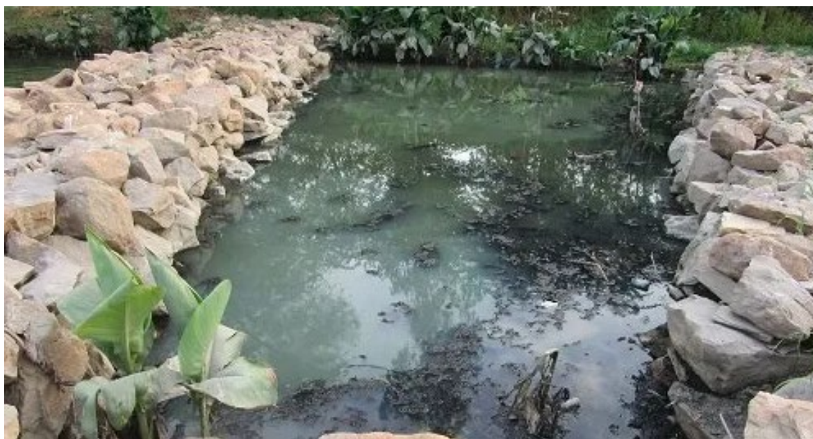
Figure 40. Application of horizontal flow filter in canal leading to Udai Sagar Lake in Udaipur (Source: Vikalpsangam)
