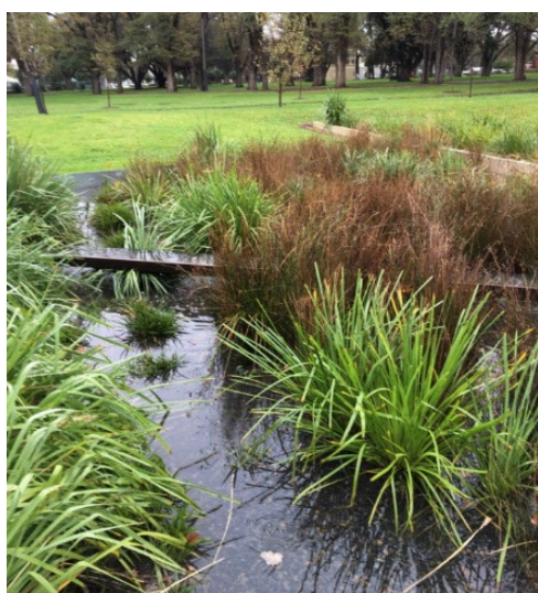
Figure 43. Application and schematic of a biofiltration system
