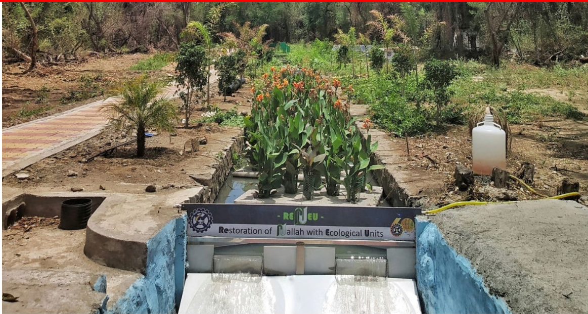
Figure 41. Installation of floating wetlands cells in a drain (Source: NEERI)
