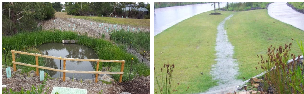
Figure 45. Pre-treatment measures for biofiltration system and other stormwater treatment assets – Sediment ponds (left) and swales (right)
