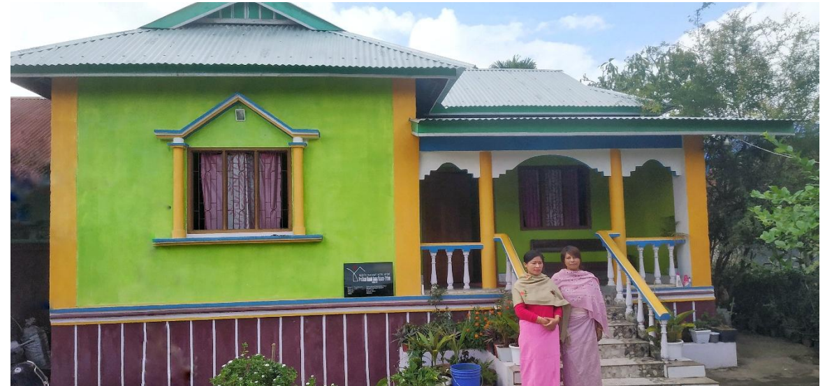
Single Family Dwelling Units
