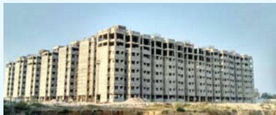
Completed project under In-Situ Slum Redevelopment of PMAY(U) in Baroda, Gujarat
