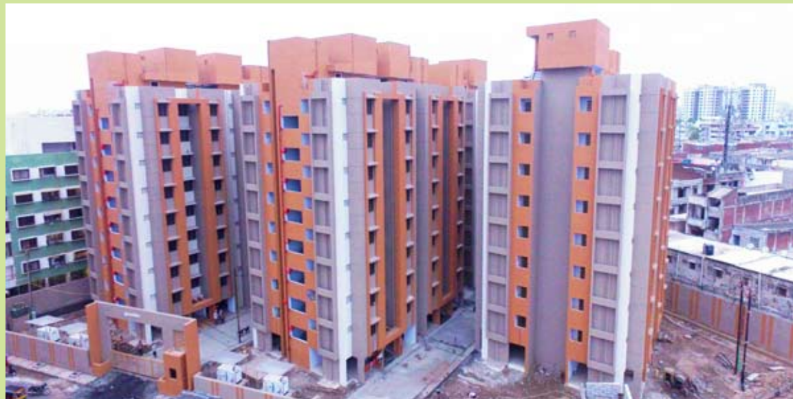
Houses constructed under AHP, Surat, Gujarat
