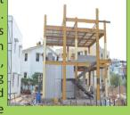
transported to the site for installation which is done using crane and other required machineries. Once all the components are assembled and erected at site, appropriate wall panels are fixed.
