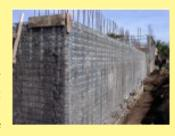
wall and slab is poured in single operation to create monolithic structure.
