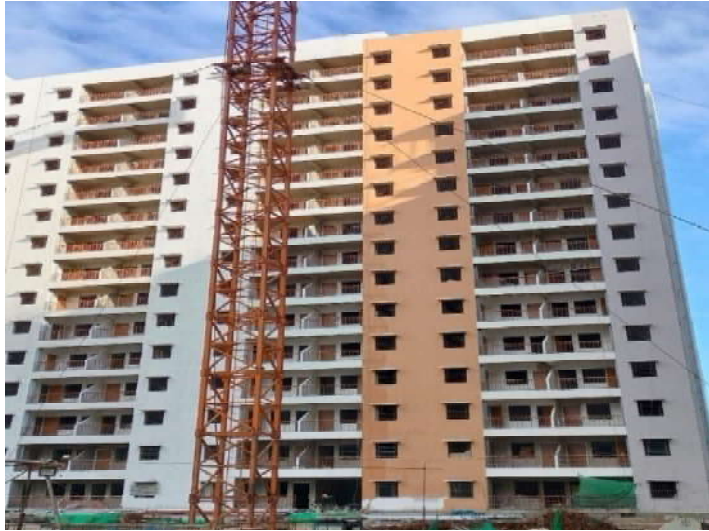
Jailorwala Bagh in-situ slum rehabilitation project
