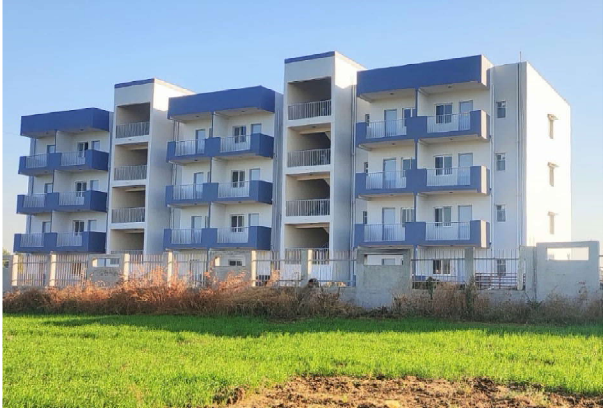
Demonstration Housing Project (Sports Hostel) under PMAY(U) completed by BMTPC using Stay-in-Place Formwork System - Insulating Concrete Forms (ICF) at Bhopal, Madhya Pradesh
