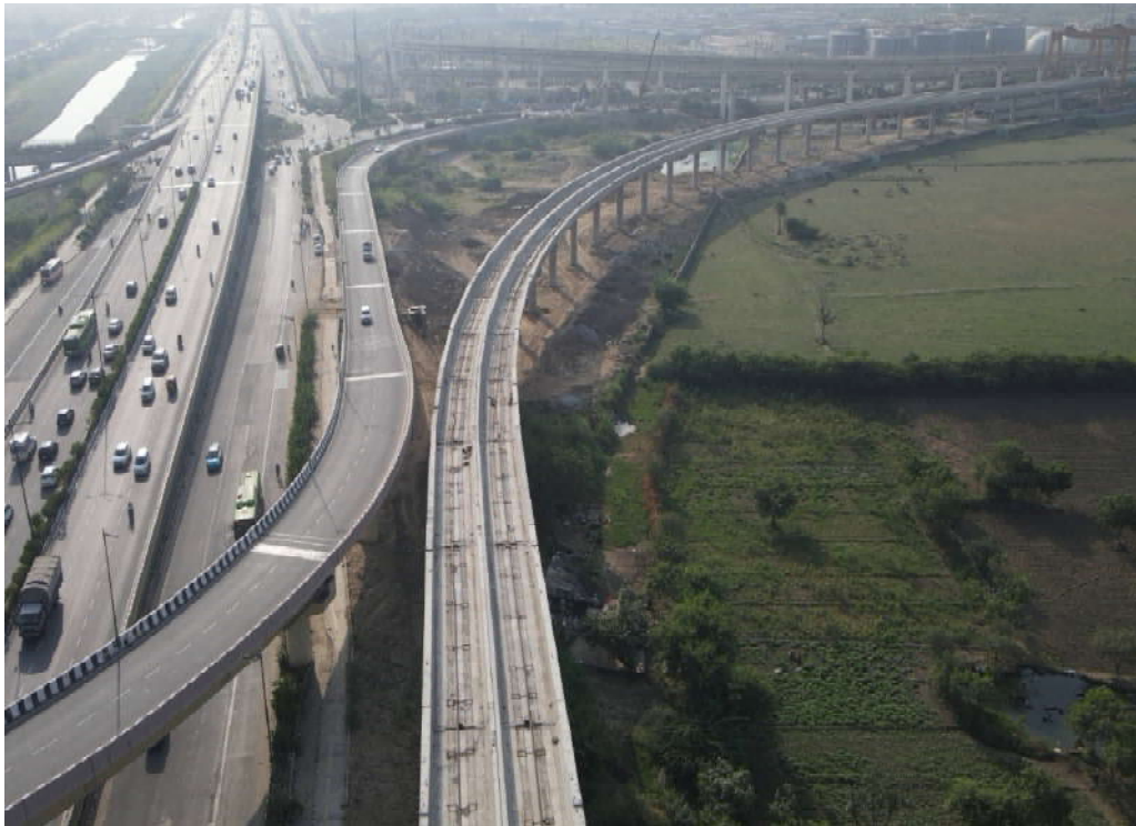
Viaduct between Mukundpur and Bhalswa
