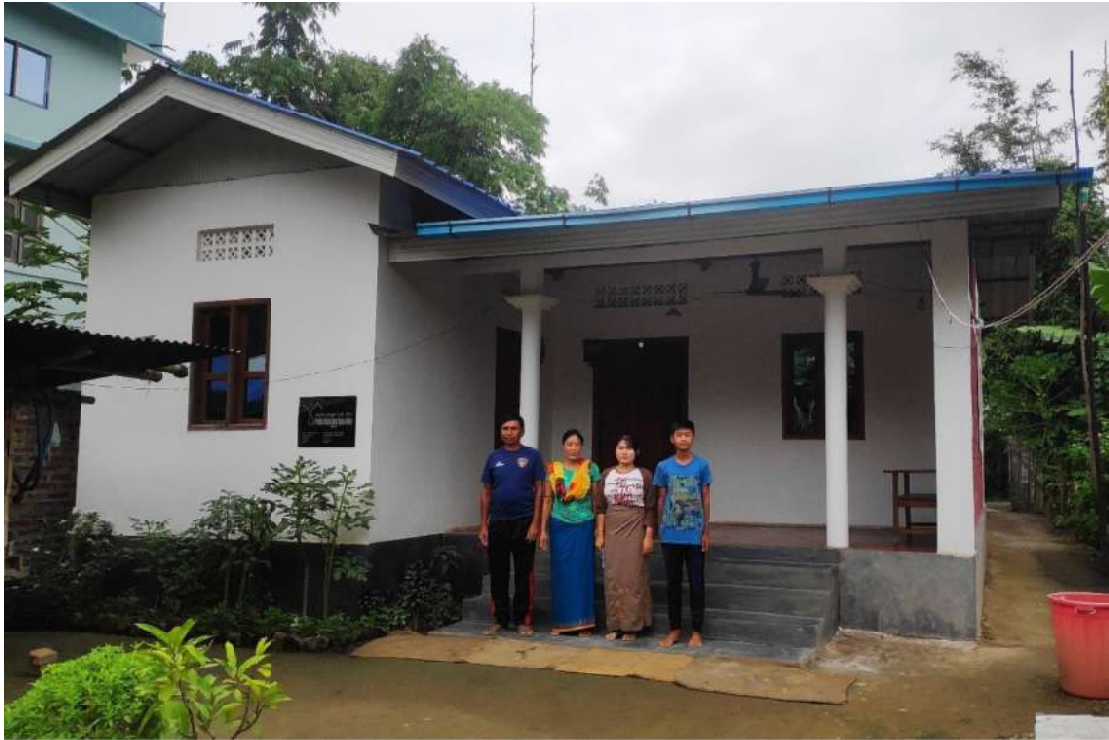
House under BLC vertical of Pradhan Mantri Awas Yojana (Urban) in Oinam, Manipur
