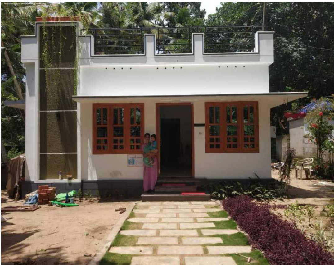
House under BLC vertical of Pradhan Mantri Awas Yojana (Urban) in Thiruvananthapuram, Kerala
