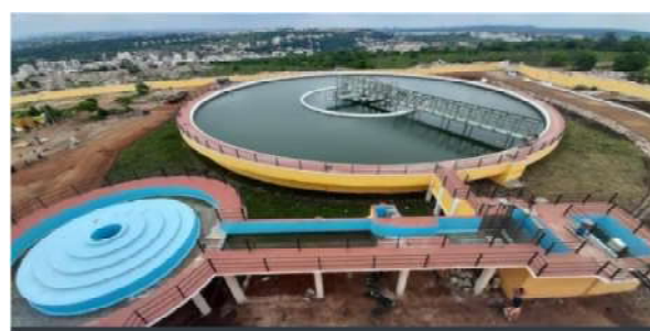
WTP at Bhopal, Madhya Pradesh
