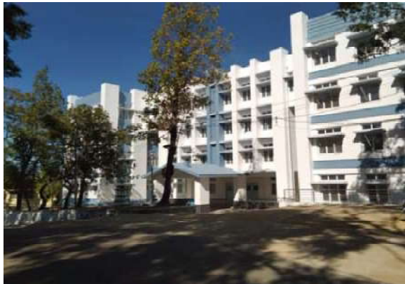
Administrative block of BSF at Frontier head quarter, Umpling, Shillong
