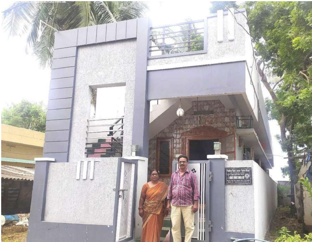
House under BLC vertical of Pradhan Mantri Awas Yojana (Urban) in Bhimavaram, Andhra Pradesh
