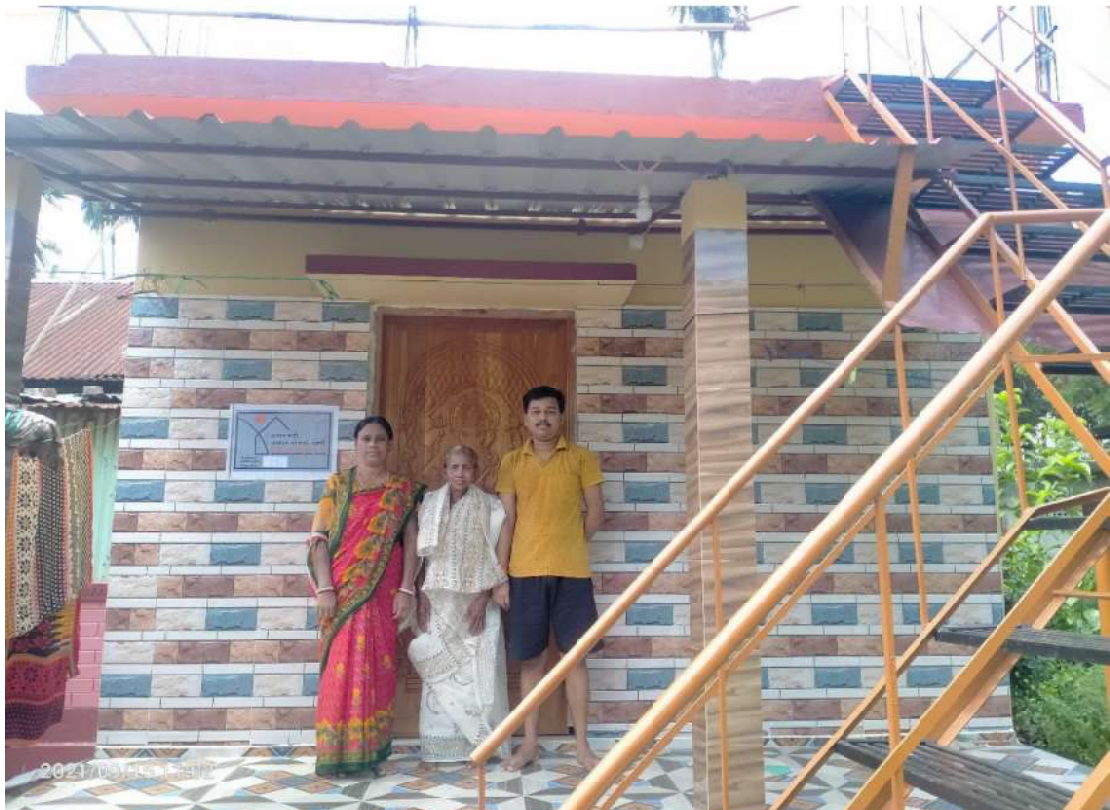
House under BLC vertical of Pradhan Mantri Awas Yojana (Urban) in Agartala, Tripura
