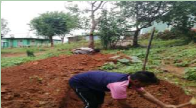
Earth Work for footing (NC) Beneficiary- Smt. Shongsuk Rympei
