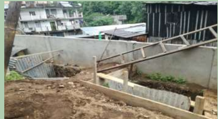
Earth Work for footing (Enhancement) Beneficiary- Smt. Shasha Lyngshing
