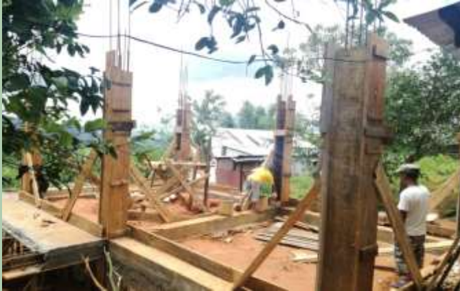
Work Completed upto Plinth Level (NC) Beneficiary- Smt. Shasha Rympei
