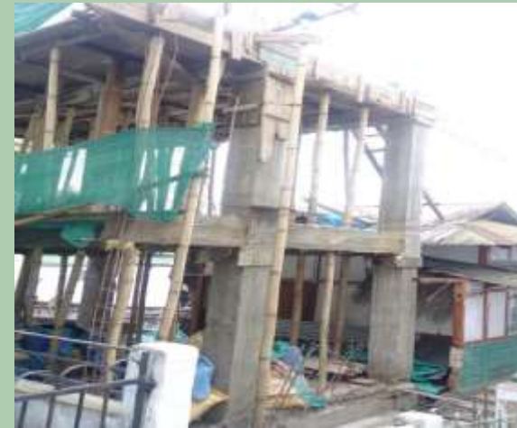
Work Completed upto Roof Level structure (NC) Beneficiary- Smt. Larihun Nongsiej
