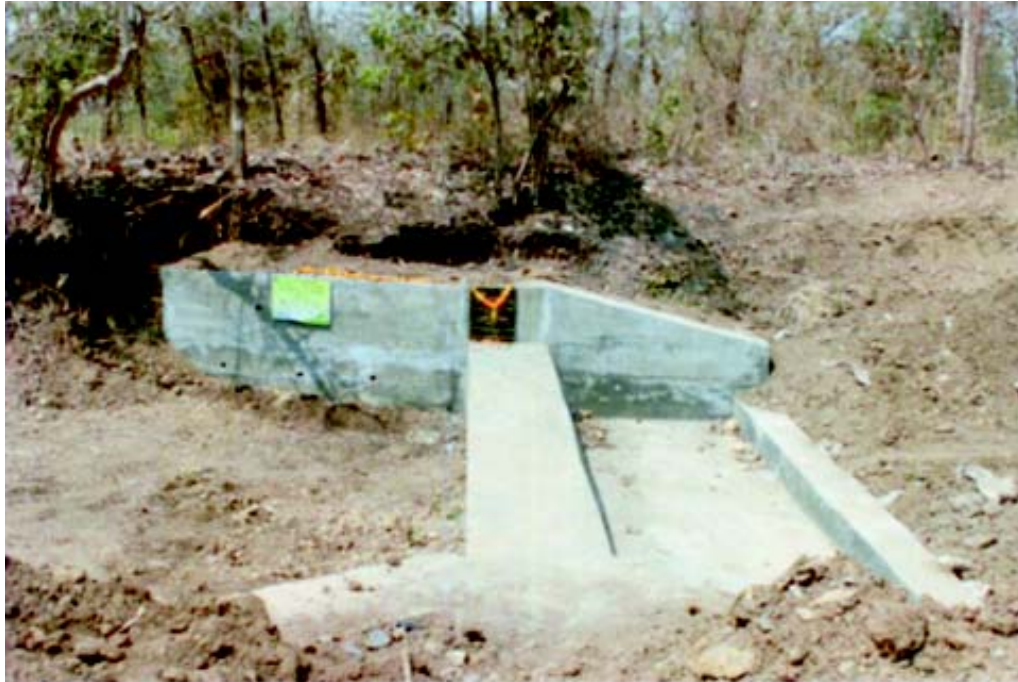
The check Dam Constructed at Village-Kusapur, Distt-Thane, Maharashtra
