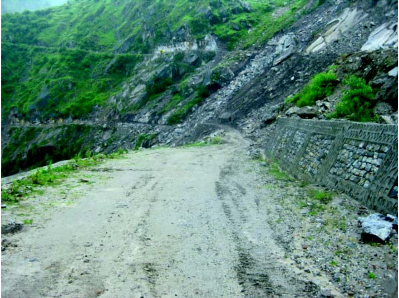
Indo China Border Road in Uttarakhand - Formation and Breast Wall constructed
