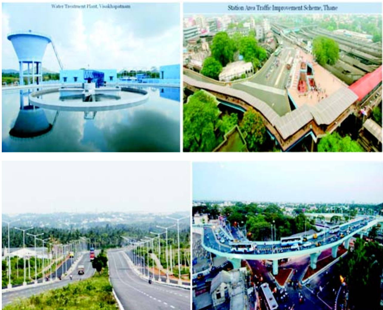
Figure 10: Glimpse of Projects completed under JnNURM
