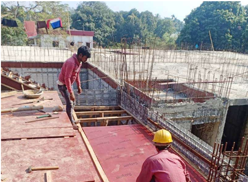
Demonstration Housing Project (Hostel for Destitute Women) under PMAY(U) being constructed by BMTPC using Structural Stay In Place Steel Formwork at Agartala, Tripura
