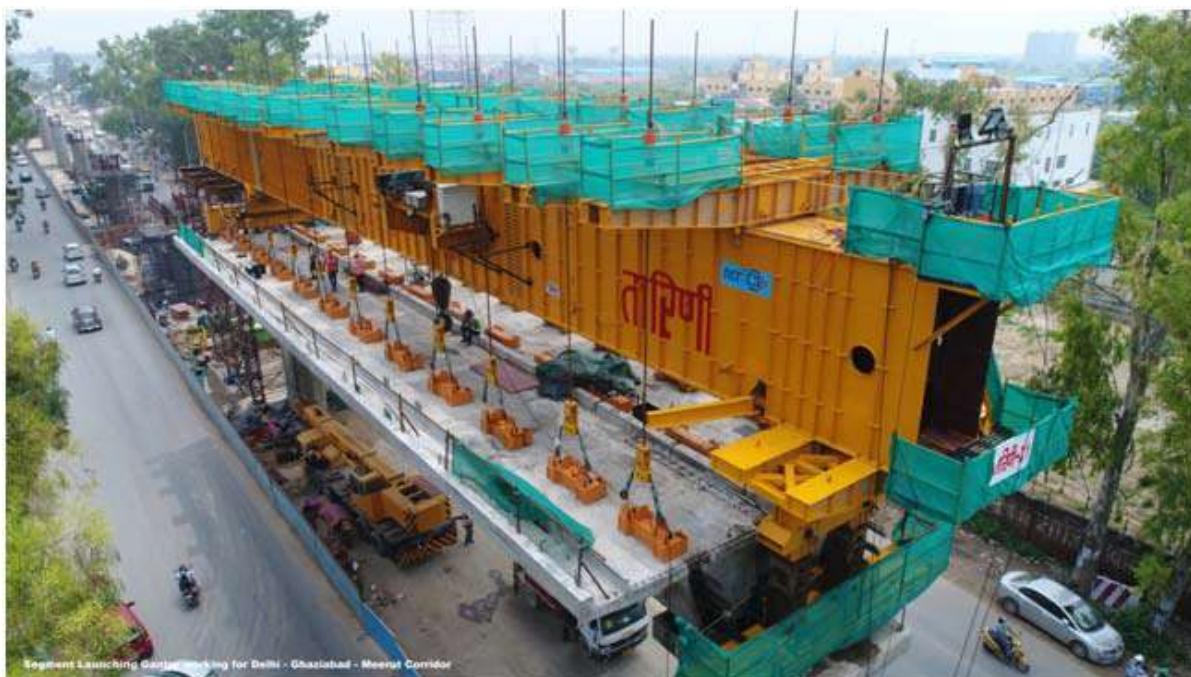
Segment Launching Gantry working for Delhi - Ghaziabad - Meerut Corridor
