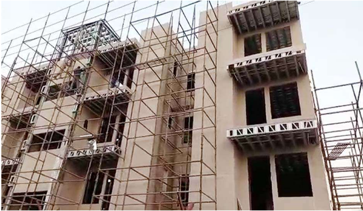
Demonstration Housing Project (Working Women Hostel) under PMAY(U) being constructed by BMTPC using Light Gauge Steel Framework System (LGSF) with Fibre Cement Board on both side and infill of rock wool at Panchkula, Haryana
