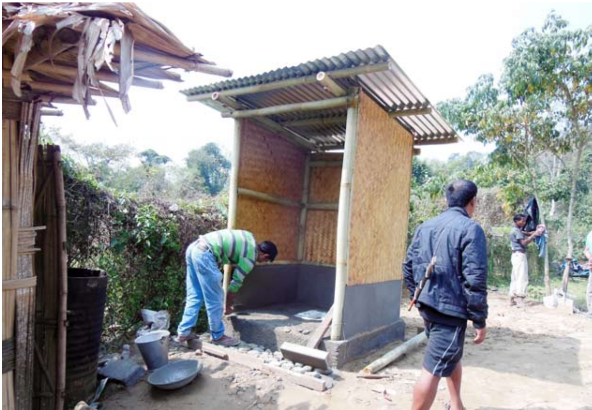
Construction of Bamboo Toilet during Training Programme on use of Bamboo in Housing and Building Construction from February 29, 2016 - March 5, 2016 at Itanagar, Arunachal Pradesh
