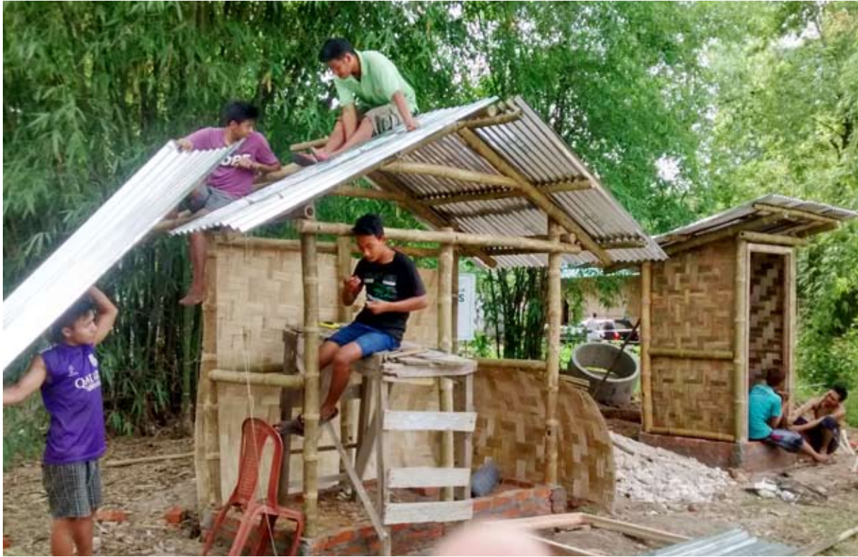
Construction of Bamboo Toilet during Training Programme on Bamboo Structure of Housing and Construction organized by BMTPC from May 12 – 16, 2015 at Dimapur, Nagaland.
