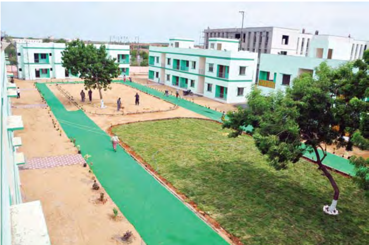
Completed Demonstration Houses at Saraswathi Nagar, Venkatachalam Mandal, SPS Nellore District, Andhra Pradesh
