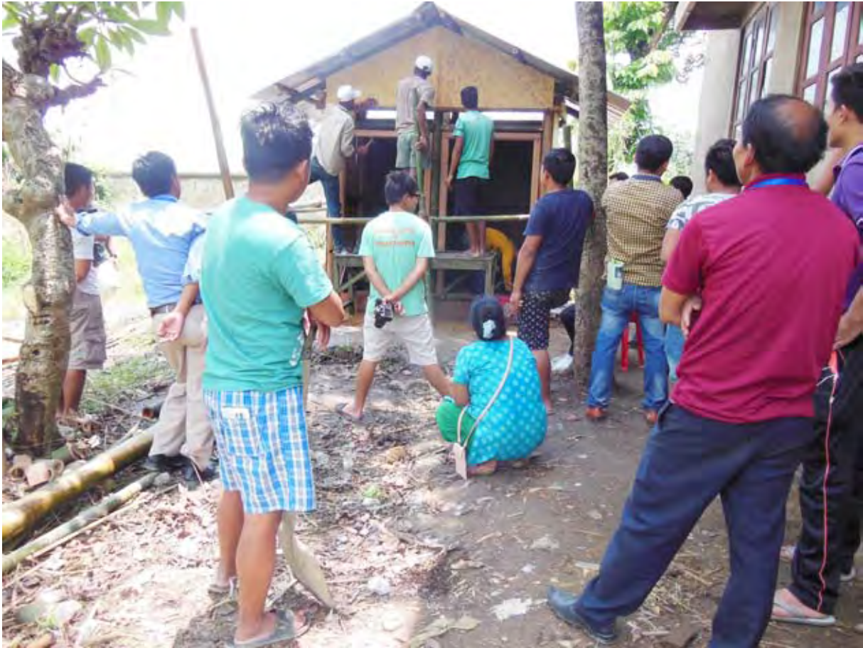
Construction of Toilet during Training Programme on “Bamboo based Toilet Building” at Imphal, Manipur from May 13-17, 2016
