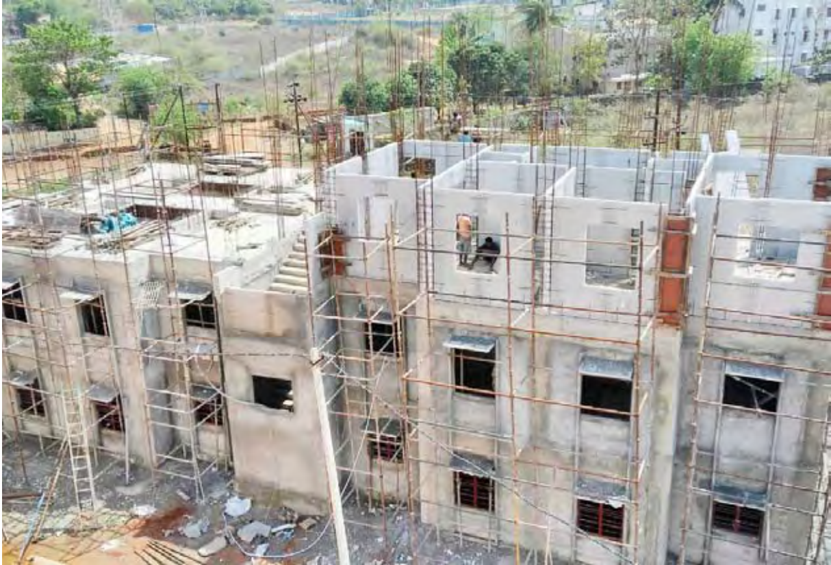
Construction of Demonstration Housing Project at Bhubaneswar, Odisha
