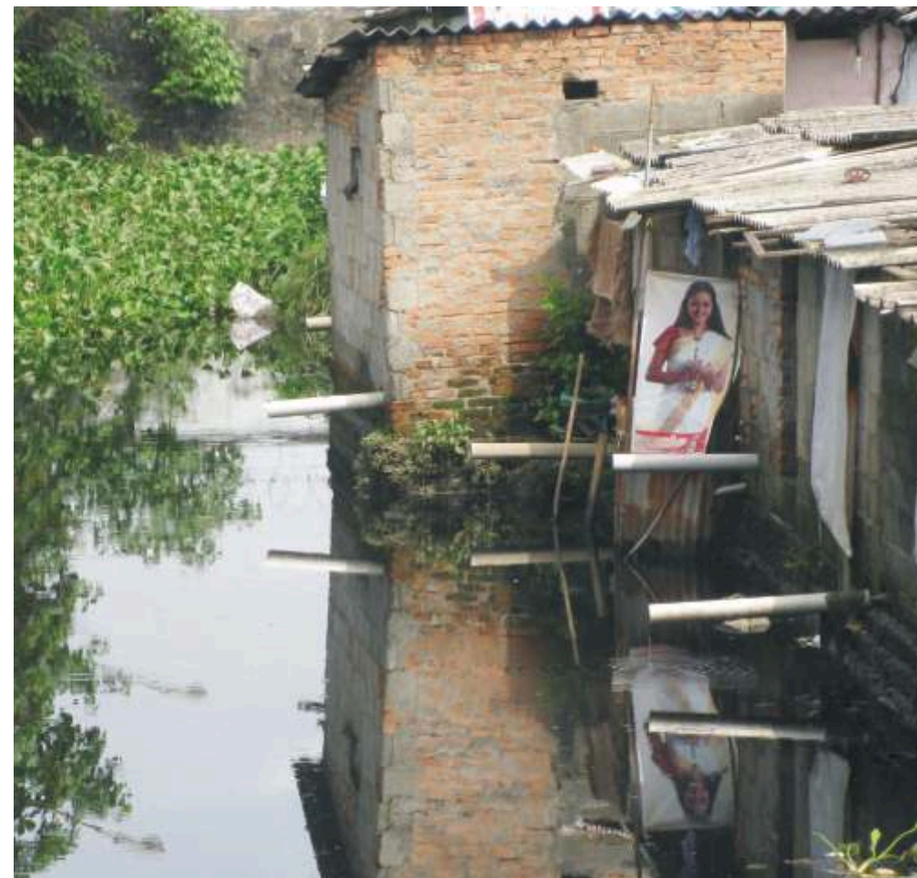
Figure 34: Clogging of storm drains
