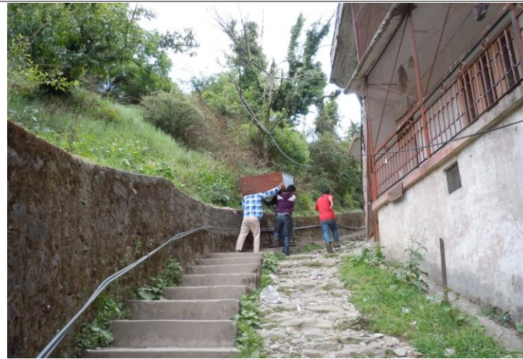
Poor conditions of pathways
