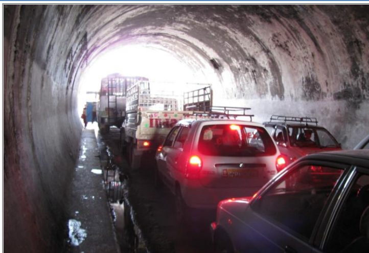
Traffic congestion inside the Victory tunnel
