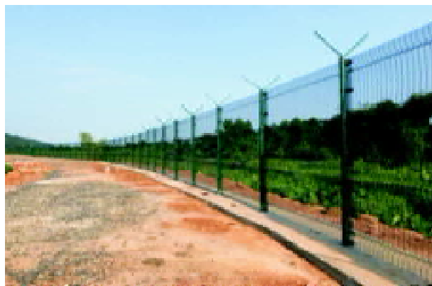
Fencing work, Meghalaya
