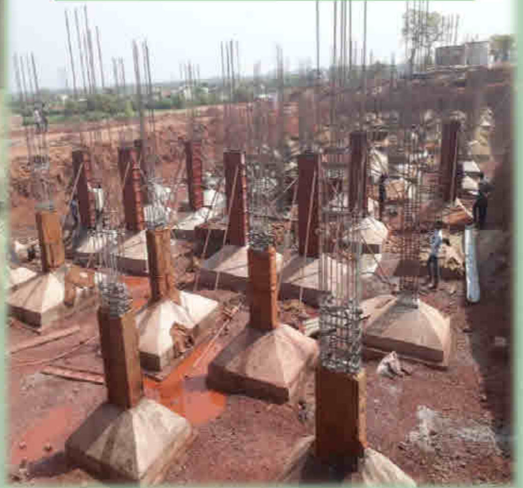
Under Construction DUs in Gwalior
