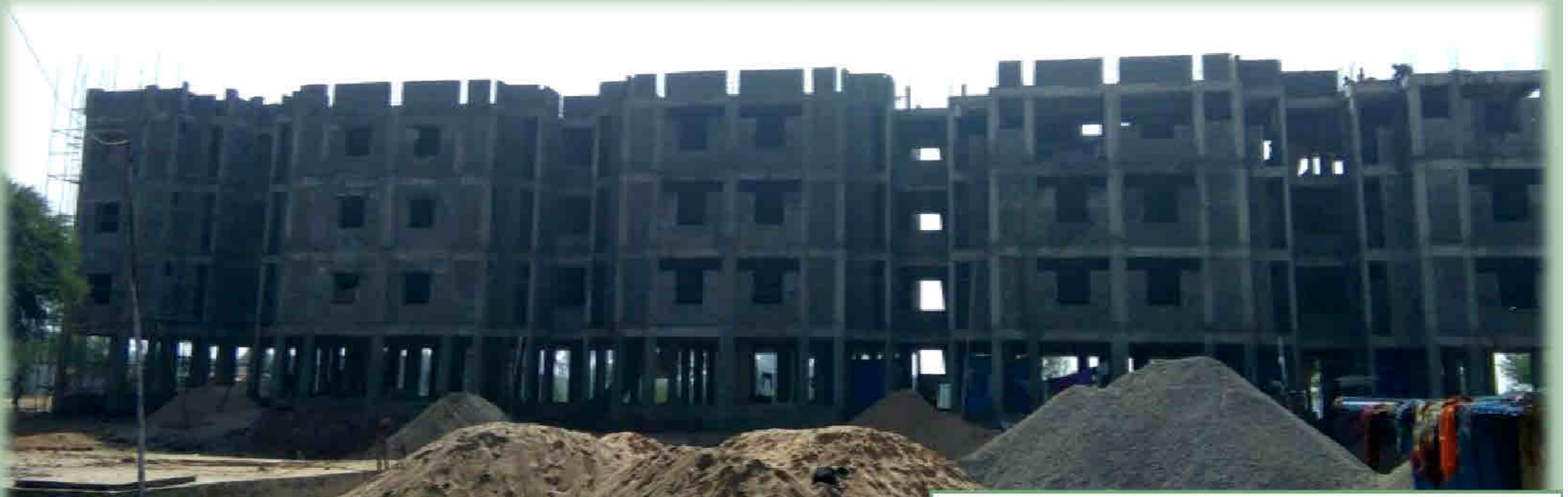
Under Construction DUs in Rewa
