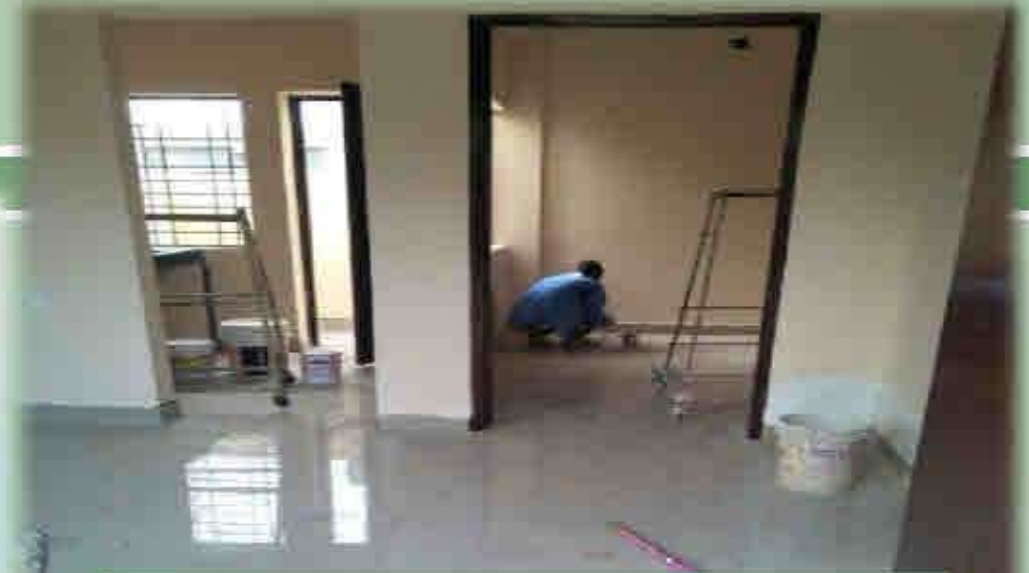
Under Construction DUs in Shahganj
