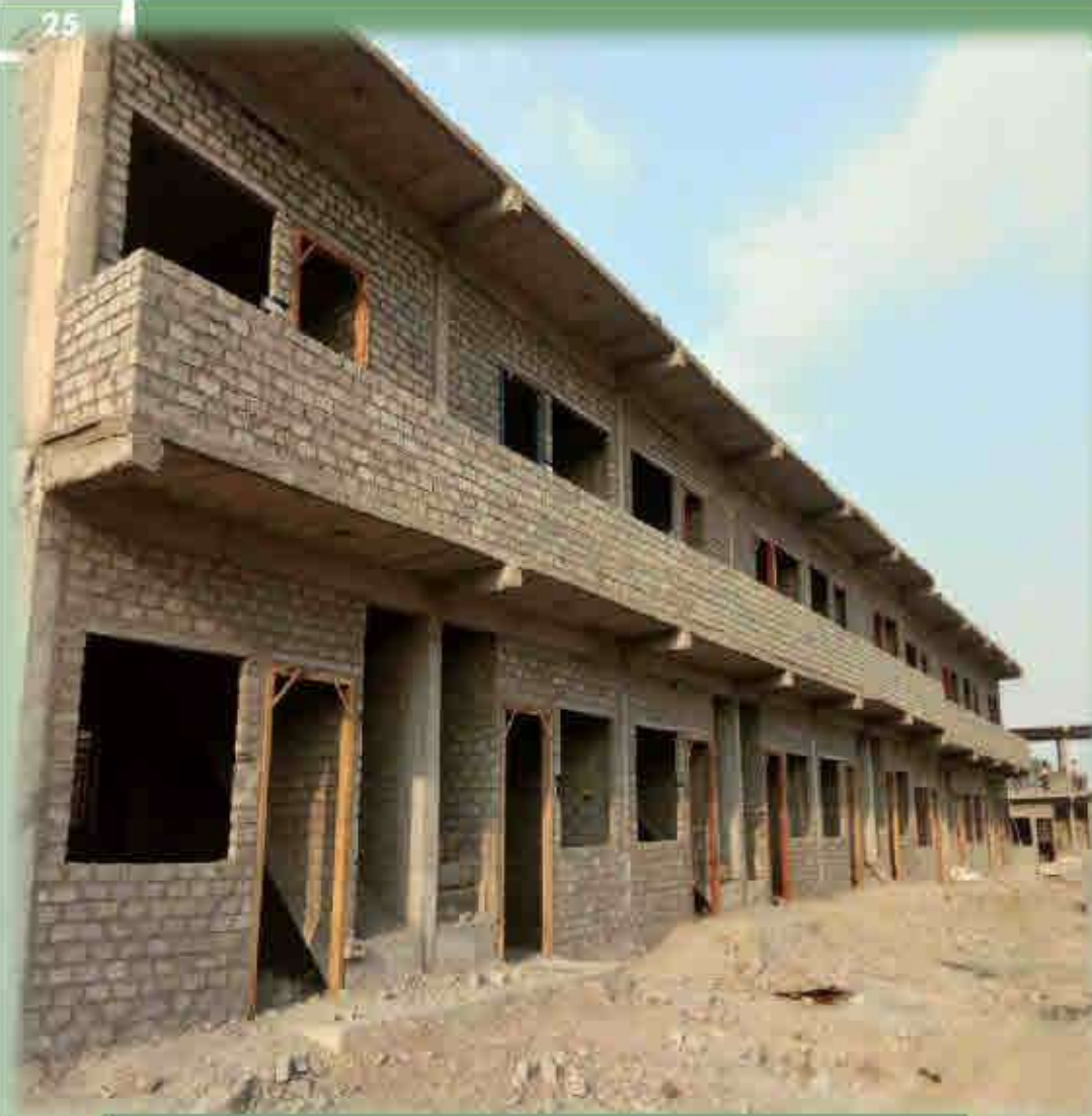
Under Construction DUs in Patharia
