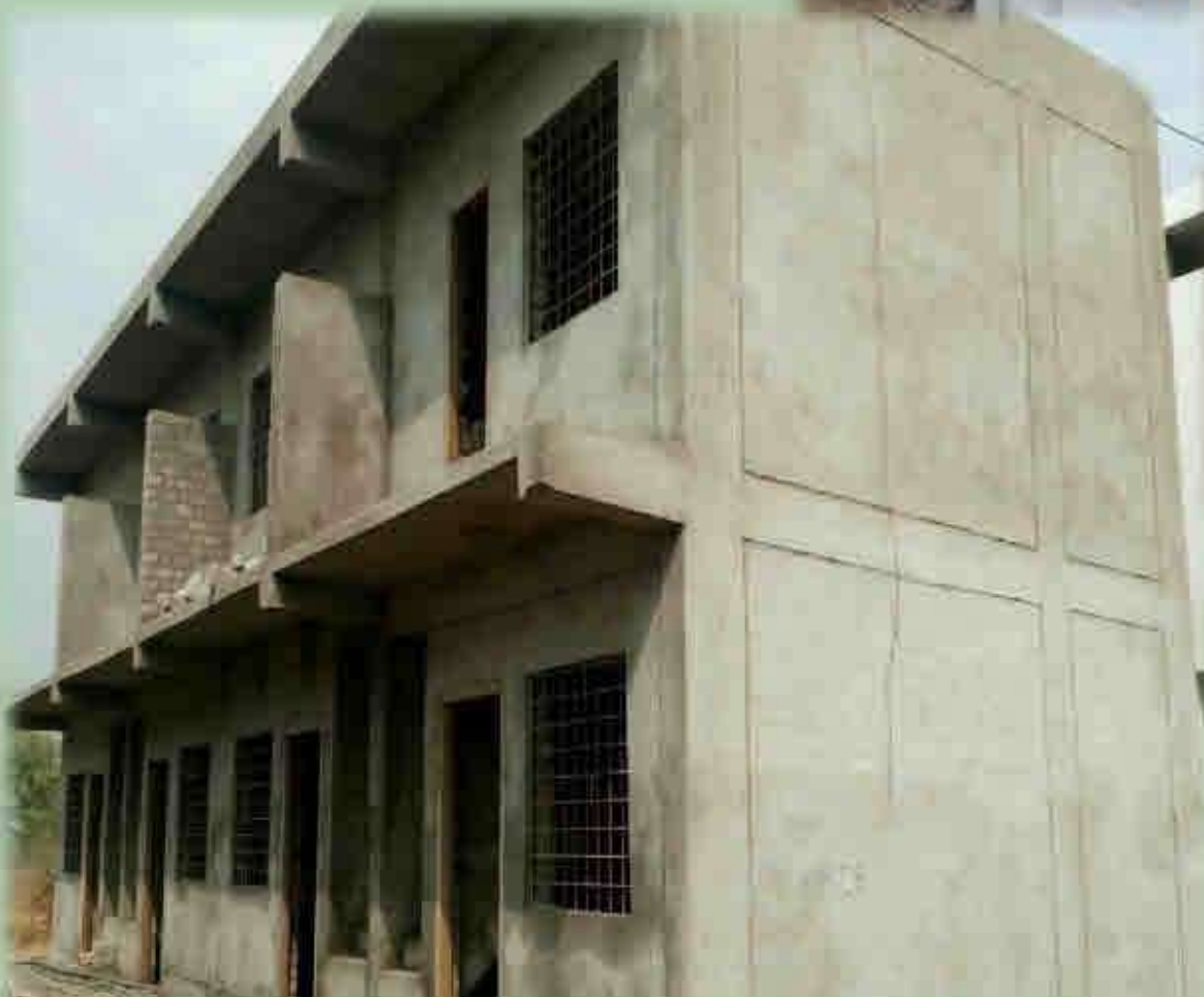
Under Construction DUs in Rampur-Baghelan
