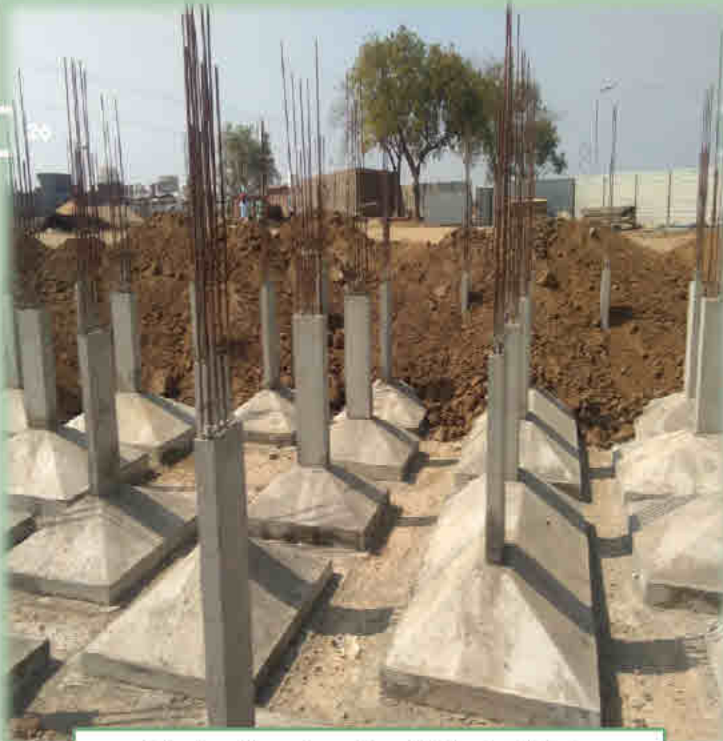
Under Construction DUs in Ujjain
