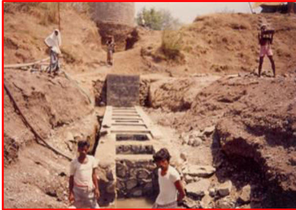
Figure 10.33: Horizontal Flow Filters
