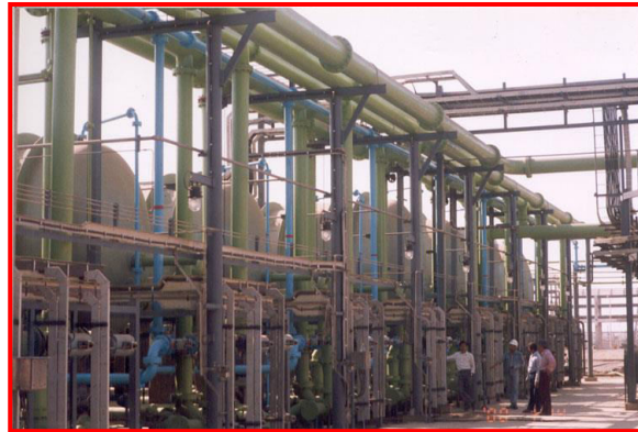
Figure: Two stage Pressure Filtration and High-Pressure Pumps and RO Skids
