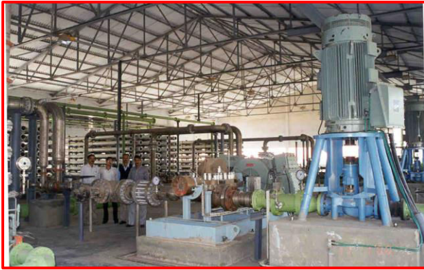
Figure: Two stage Pressure Filtration and High-Pressure Pumps and RO Skids
