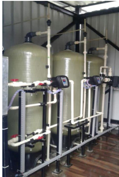
Figure 10.5: IRP Plant with Auto Multiport Valve
