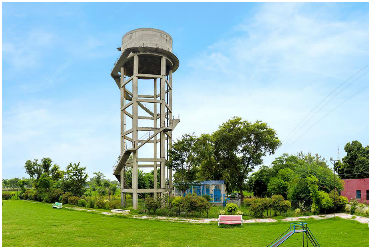
Figure 10.9 A typical iron and arsenic removal community water treatment plant in Punjab. The installation was done by Hydro-materials Pvt. Ltd., an IIT Madras incubated company. The blue-colored unit, below the overhead tank, is the purification unit and the treated water is distributed to the village
