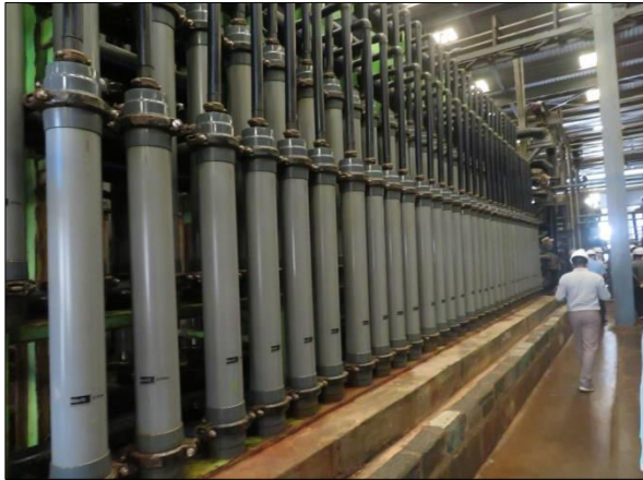
Figure 10.31: UF Membranes Skids
