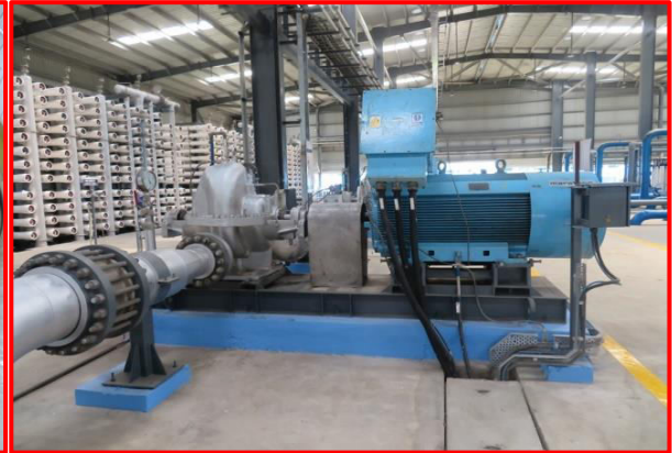
Figure 10.26: High-Pressure RO feed Pump
