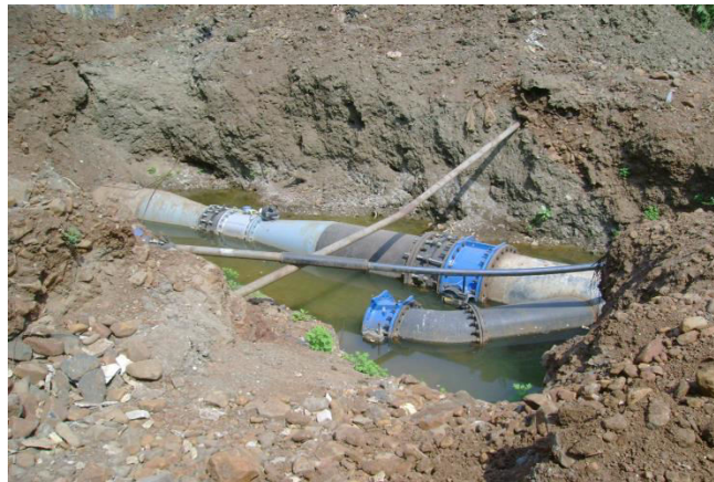
Figure 3: Replacement of leaking valve (an example of control measure implementation)
