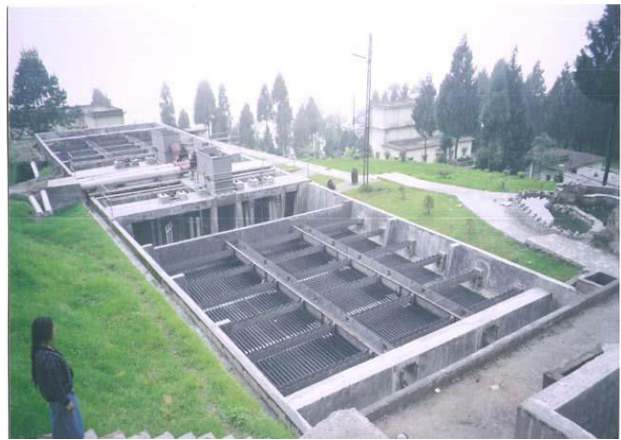
Figure 8.95: Retrofitting of a rectangular tank with tube settler (Selep, Gangtok, Sikkim)
