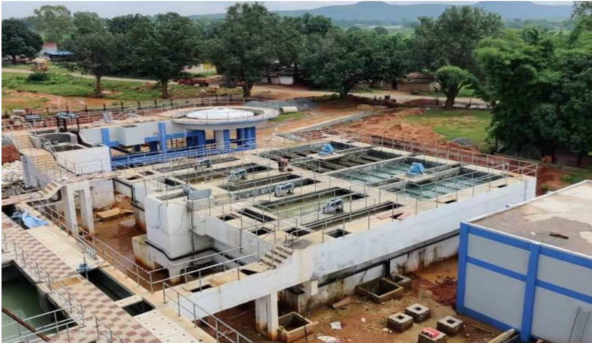
Figure 8.36: WTP at Ambikapur, Madhya Pradesh, Capacity 18 mld with External flocculators and Tube Settling Tank with Central Rake
