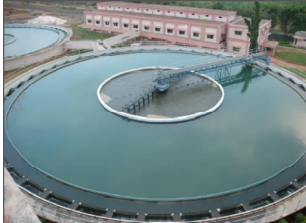
Figure 8.97: Upgraded 75 MLD WTP to 123 MLD at Madurai by inserting tube settlers in clarifier rims and changeover of RSFs to Dual Media Filters
