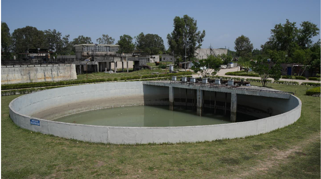
Figure 8.77: Wash Water Recycle Tanks
