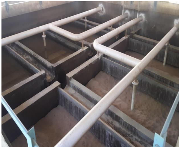
Figure 8.71: MMDB filters at Pench PH-II, Nagpur
