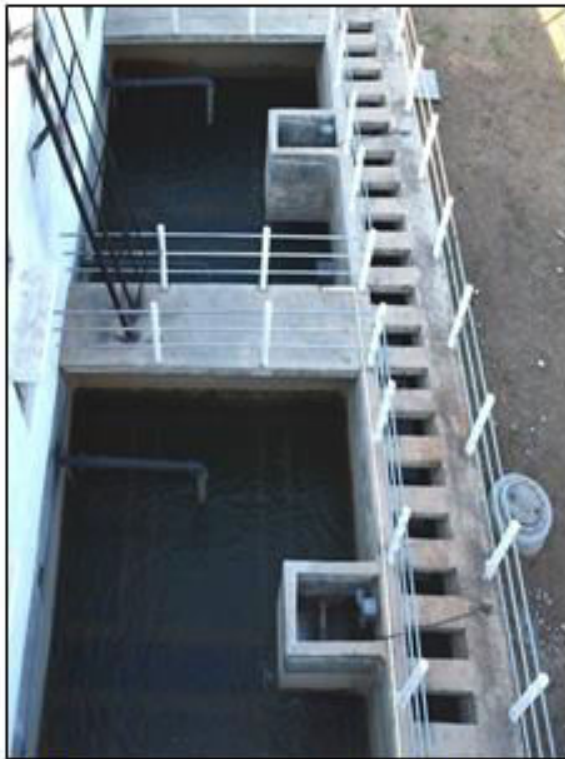
Filter Inlet Channel and Inlet Weir with chambers
