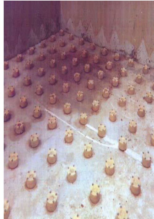
Figure 8.56: Finished Filter floor after erection of nozzles
