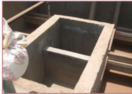
Close-up of splitter weir and Chamber
