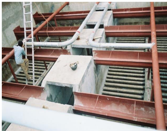
Figure 8.69: Checking media expansion during backwash using sand expansion stick
