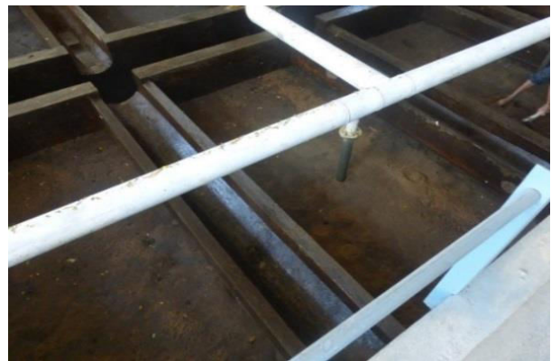
Figure 8.96: Upgrading of Existing conventional filter beds with mono media deep bed filters (Pench II, OCW, Nagpur)
