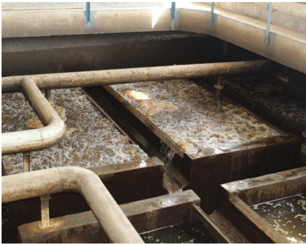
Figure 8.61: Filter bed under air-scour operation
