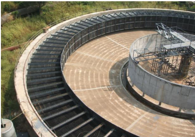
Figure 8.94: Augmentation of clariflocculator by installation of Tube Modules installed (Navi Mumbai, Maharashtra)
