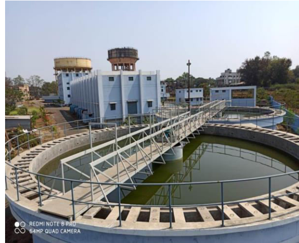
Figure 8.81: Picture of a Sludge Thickener (Source – Sangli, Maharashtra)
