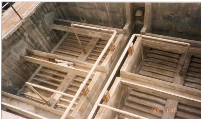
Figure 8.51: Perforated Pipe Under-drain
