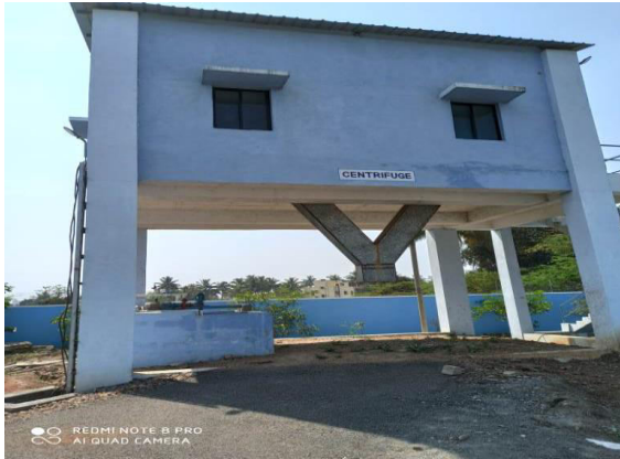
Figure 8.85: Centrifuge Building with “chute” (source- Sangli, Maharashtra)
