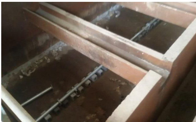
Figure 8.96: Upgrading of Existing conventional filter beds with mono media deep bed filters (Pench II, OCW, Nagpur)
