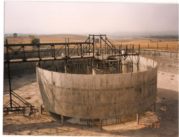
Figure 8.18: Flocculation zone with slow agitators
