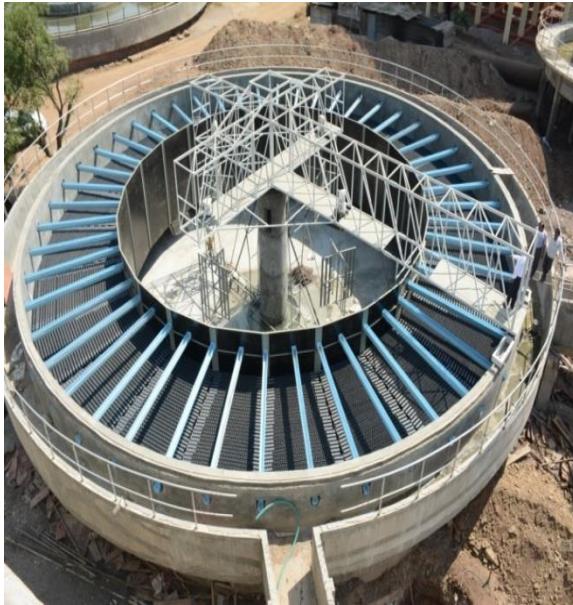
Figure 8.24: Clarisettler with Rotating Scrapper Bridge
