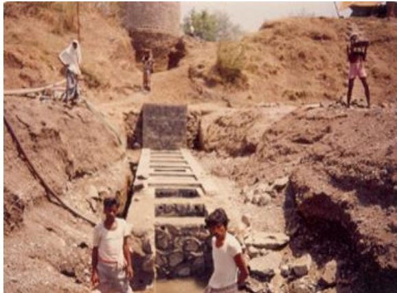
Figure 10.23: Horizontal Flow Filters
