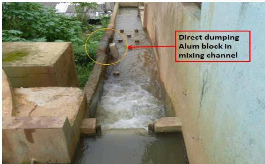
Figure 8.5: Direct dumping Alum block (Not Recommended)
