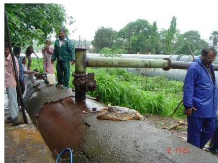
(a) 300 mm connection taken from MIDC pipeline (b) MIDC pipeline joined to MJP pipeline
