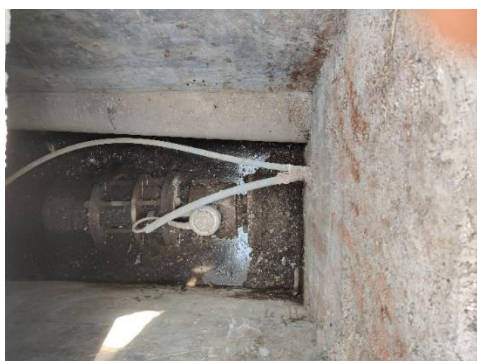
Figure 1: Bulk meters with sensor at entry of DMA
