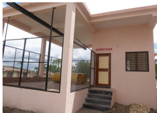
Figure 9.8: Chlorination Room and tonner yard at Ghulewadi (10 MLD) WTP, Dist. Ahemadnagar, Maharashtra
