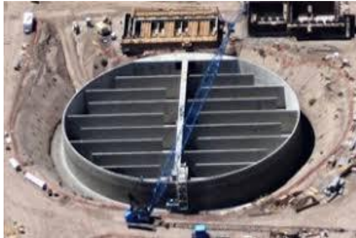
Figure 9.13: Circular contact tank under construction
