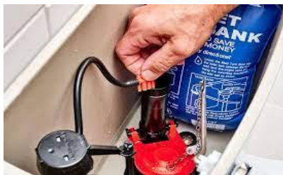
Figure 15.4: Tank bank to save on Toilet flushing
