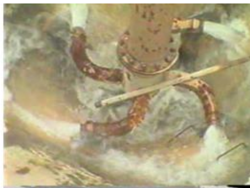
Figure 8.31: Water Jets at the Bottom of the Hopper
