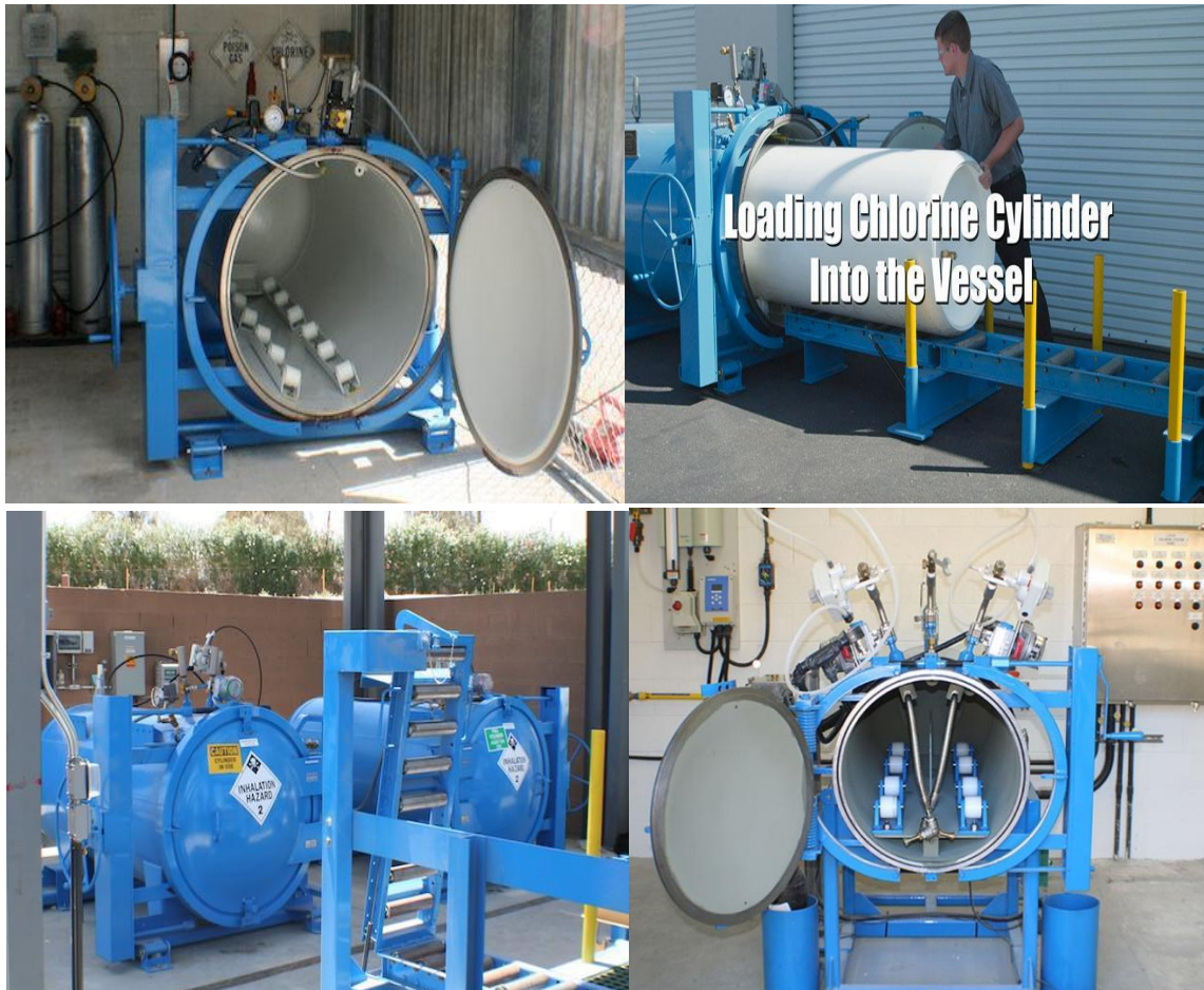
Figure 9.6: New Development as tonner safety container shells have been developed
