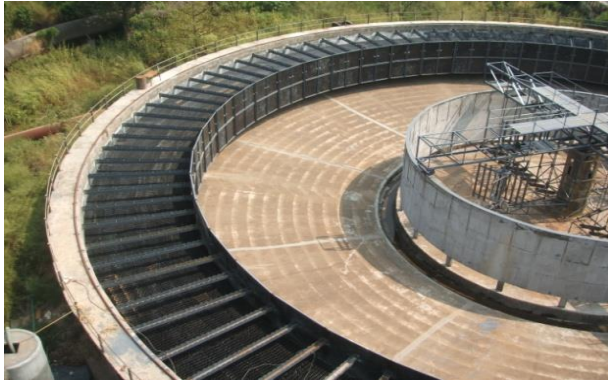
Figure 8.56: Tube Modules installed in Clariflocculator
