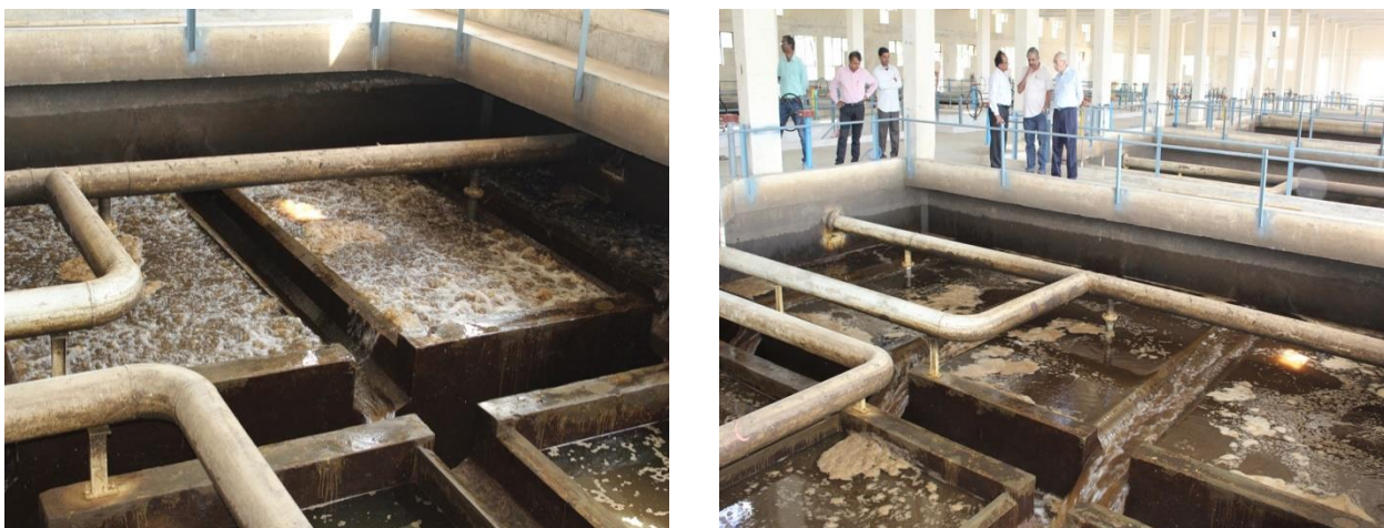
Figure 8.35: Cross-Troughs and Central gutter
