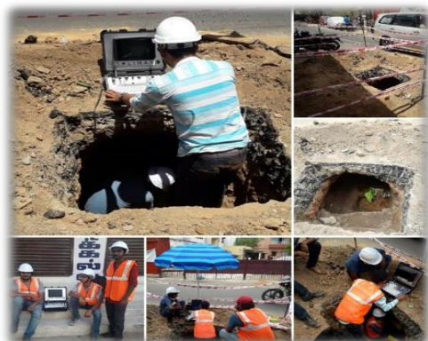
Figure 1: Glimpses of the site preparation for launching the inspection equipment.
