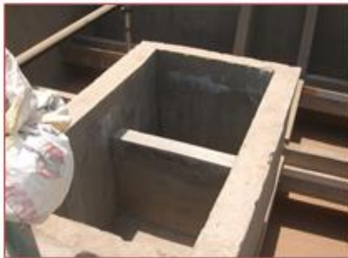
Figure 8.46: Close-up of Splitter Weir and Chamber
