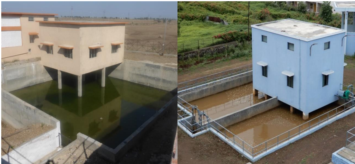
Figure 8.49: Wash Water Recycle Tanks (Single Compartment and Two Compartments)
