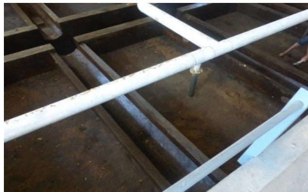
Figure 8.58: Upgrading of Existing conventional filter beds with mono media deep bed filters
