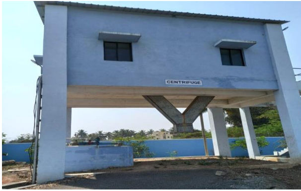
Figure 8.50: Centrifuge Building with “Chute”
