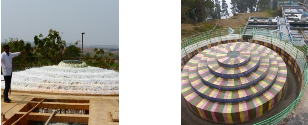
Figure 8.1: Cascade Aerators with Four to Six Steps
