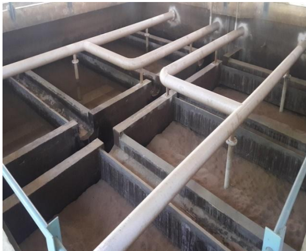
Figure 8.41: MMDB Filters
