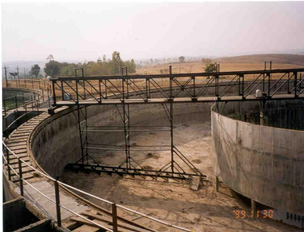
Figure 8.17: Clarification zone with scraper rotating bridge
