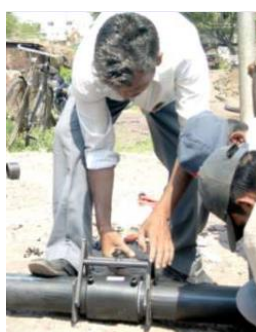
Figure 2: Jointing of pipes by electrofusion coupler
