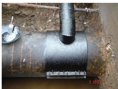
(a) 300 mm connection taken from MIDC pipeline (b) MIDC pipeline joined to MJP pipeline
