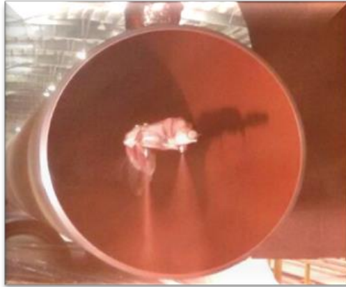
Figure 11.10: Hot airless spray of Food grade epoxy lining inside pipeline
