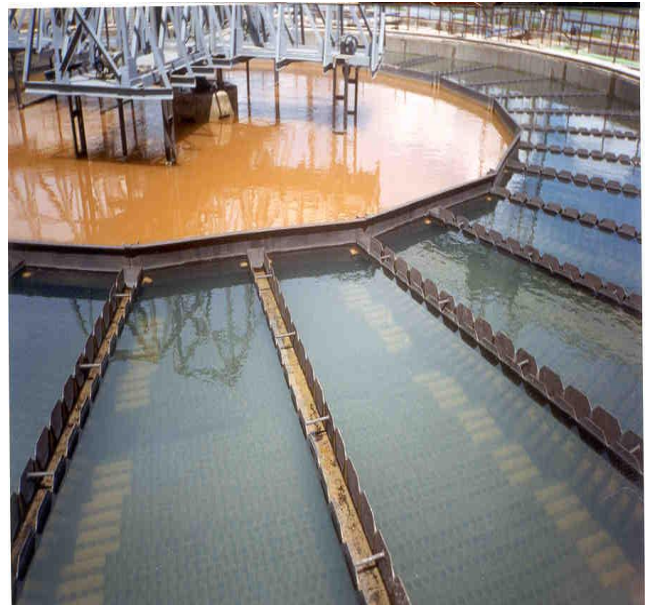
Figure 8.25: Clarisettler with Central Rake
