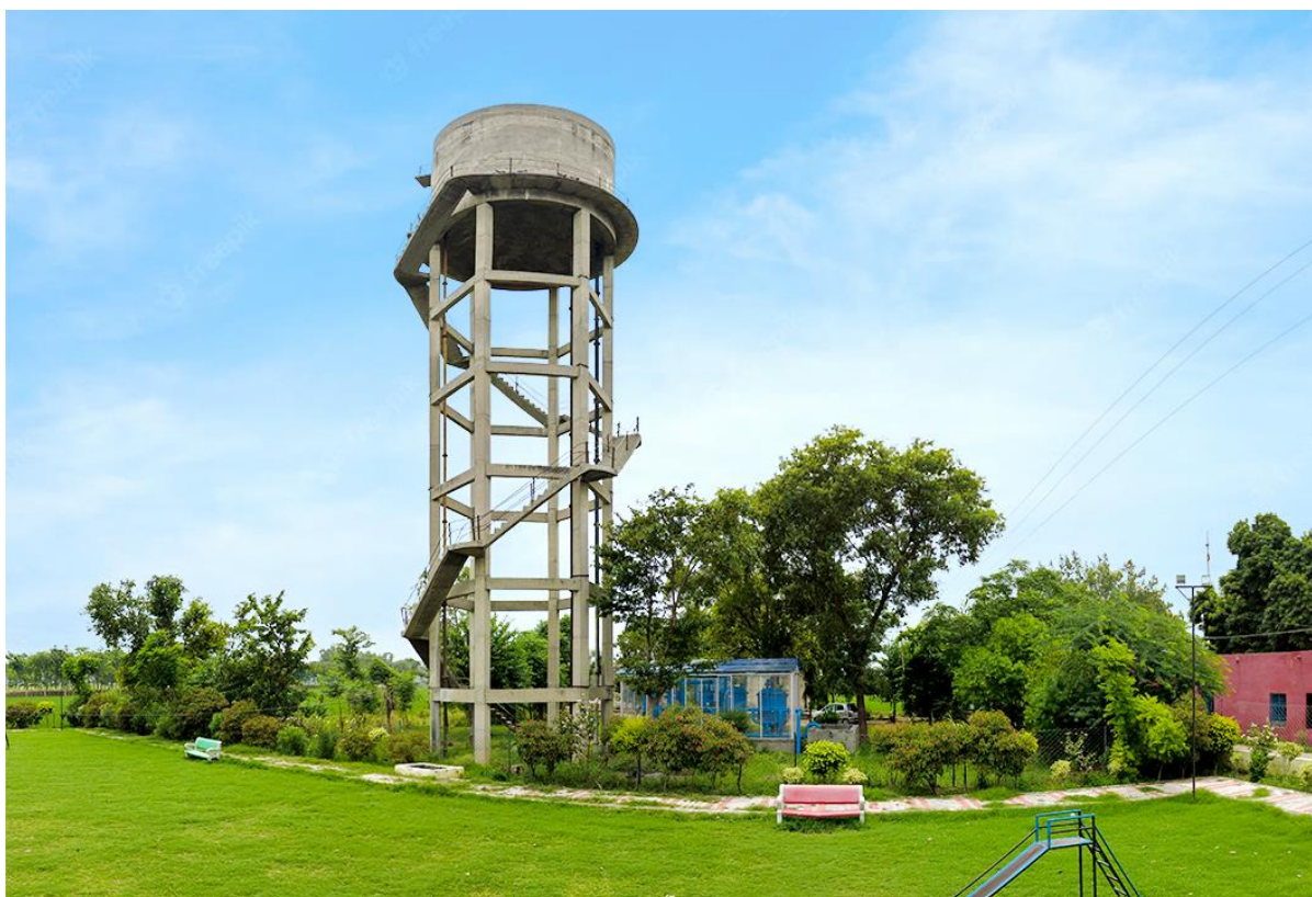
Figure 10.7: A typical iron and arsenic removal community WTP in Punjab. The blue-coloured unit, below the overhead tank, is the purification unit and the treated water is distributed to the village.
