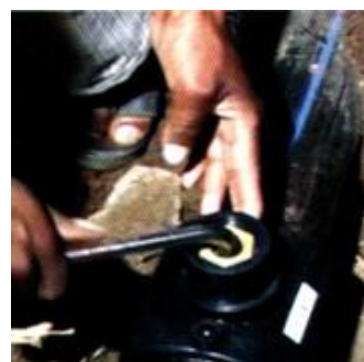
Figure 6: Consumer connection by MDPE pipe
