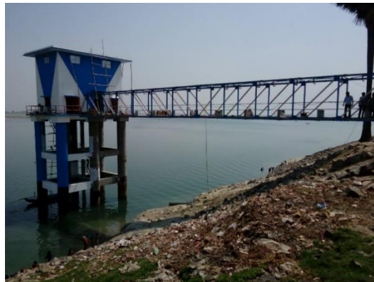
Figure 4.7: Fixed Jetty Intake
