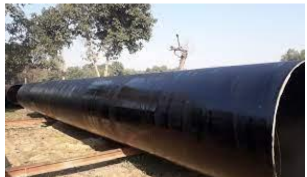
Figure 11.9: Application of tape coating in pipeline
