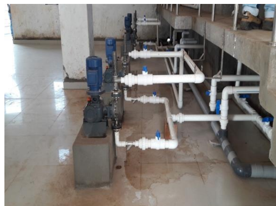
Figure 8.8: Reciprocating / Positive Displacement Pump Chemical Feeders
