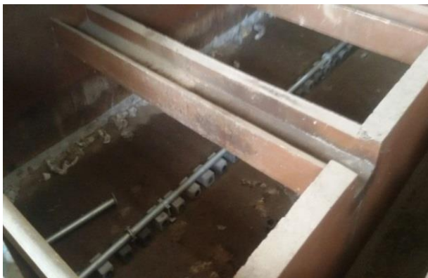
Figure 8.58: Upgrading of Existing conventional filter beds with mono media deep bed filters
