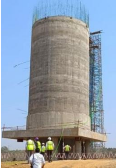
Figure 6.19: 23 m high BPT nearing Completion
