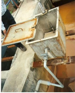
Figure 8.6: Gravity Orifice & Taper valve Dosing Box
