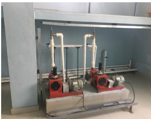
Figure 8.8: Reciprocating / Positive Displacement Pump Chemical Feeders
