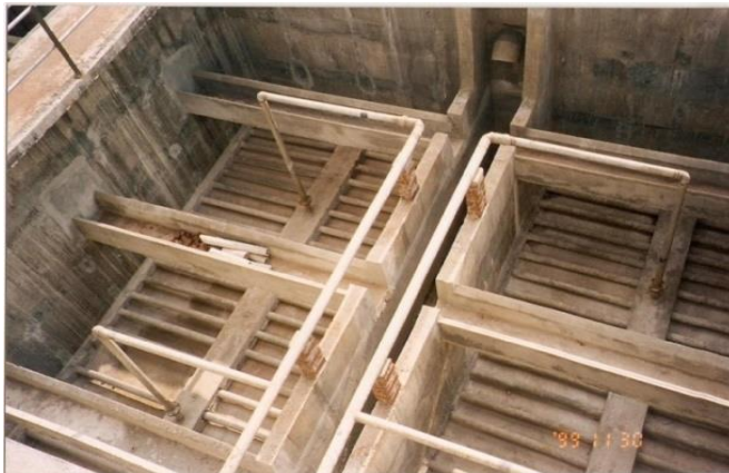
Figure 8.33: Manifold-Laterals Assembly
