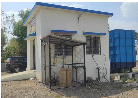
Figure 9.7: Installation of chlorine cylinders (100 kg) and chlorinators At Packaged water treatment plant, Rajapur, Dist. Ahemadnagar, Maharashtra
