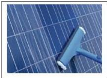
Figure 9.4: Cleaning of Panels
