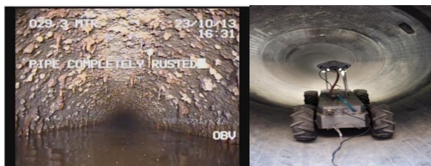
Figure 7.1: Robotic Water Pipeline Conditional Assessment
