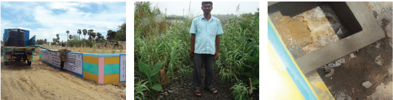
FIGURE 3.5: Sludge Treatment Plant at Musiri, Tamilnadu
