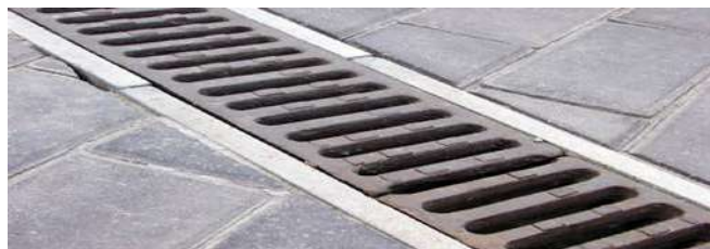
Figure 6.10:Trench Drain
