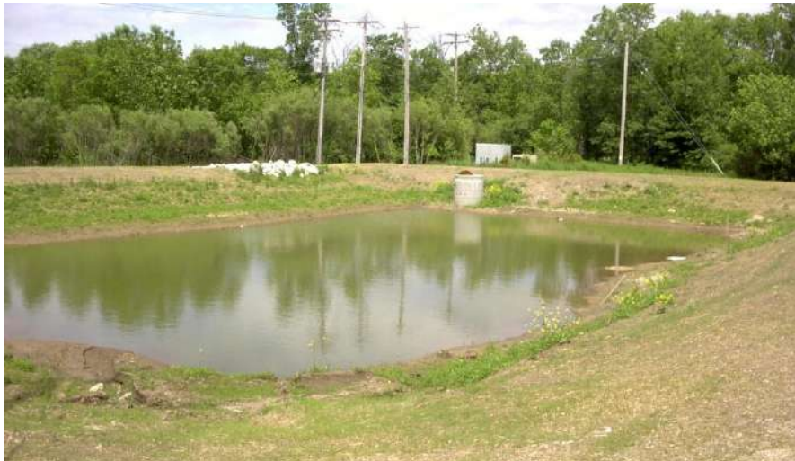
Figure 6.4: Sediment Basins
