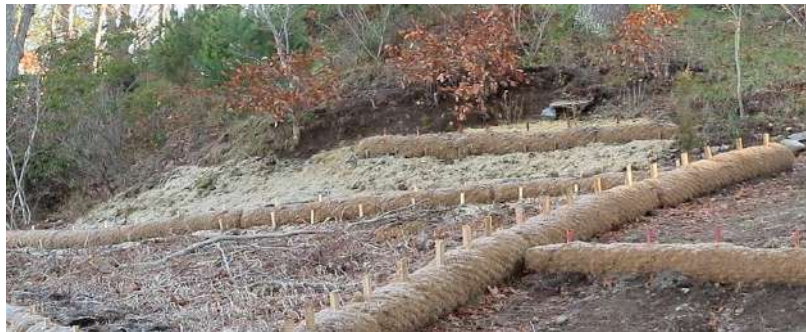
Figure 6.7: Brush Barrier
