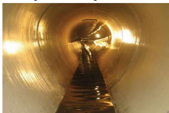
Figure 1.3: Rehabilitation of Brick Combined Sewer in Kolkata
