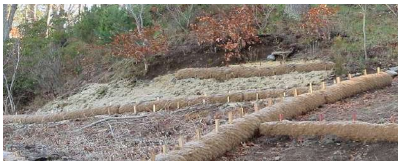
Figure 6.7: Brush Barrier
