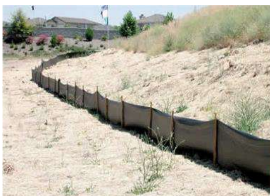
Figure 6. 6: Silt Fence
