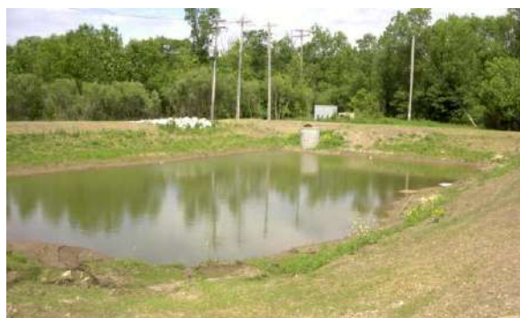
Figure 6. 4: Sediment Basin
