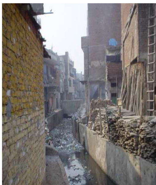
Figure 1.4: Encroachment in storm water drains
