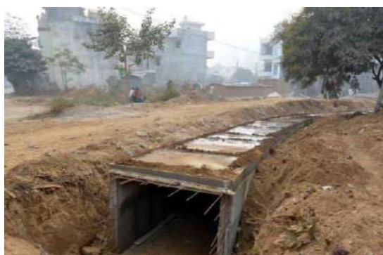
Figure 11. 7: Box drain
