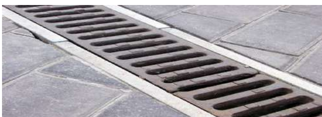
Figure 6.10: Trench Drain
