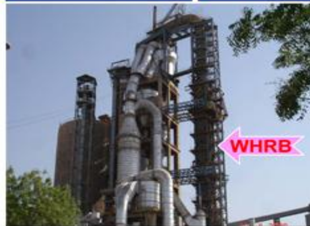
After installation of WHRB
