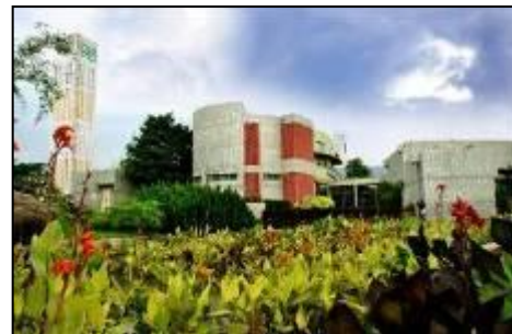
Root Zone Treatment System
