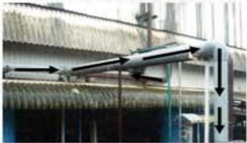
Collection of water of roof area 20 M X 15 M
