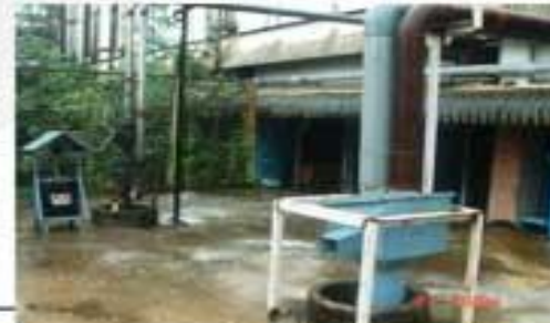
Water tank view
