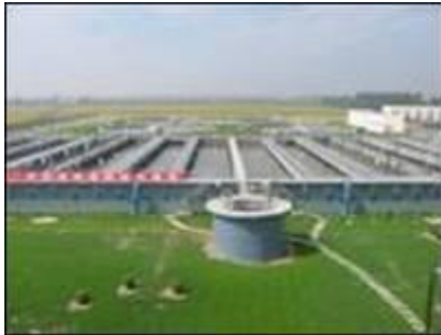
On-site Waste Water Treatment Plant
