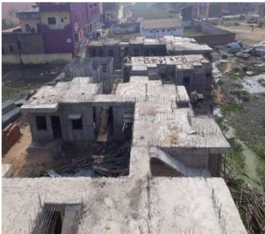
Demonstration Houses being constructed using Coffor Structural Stay in Place Formwork System by BMTPC at Bihar Shariff, Bihar
