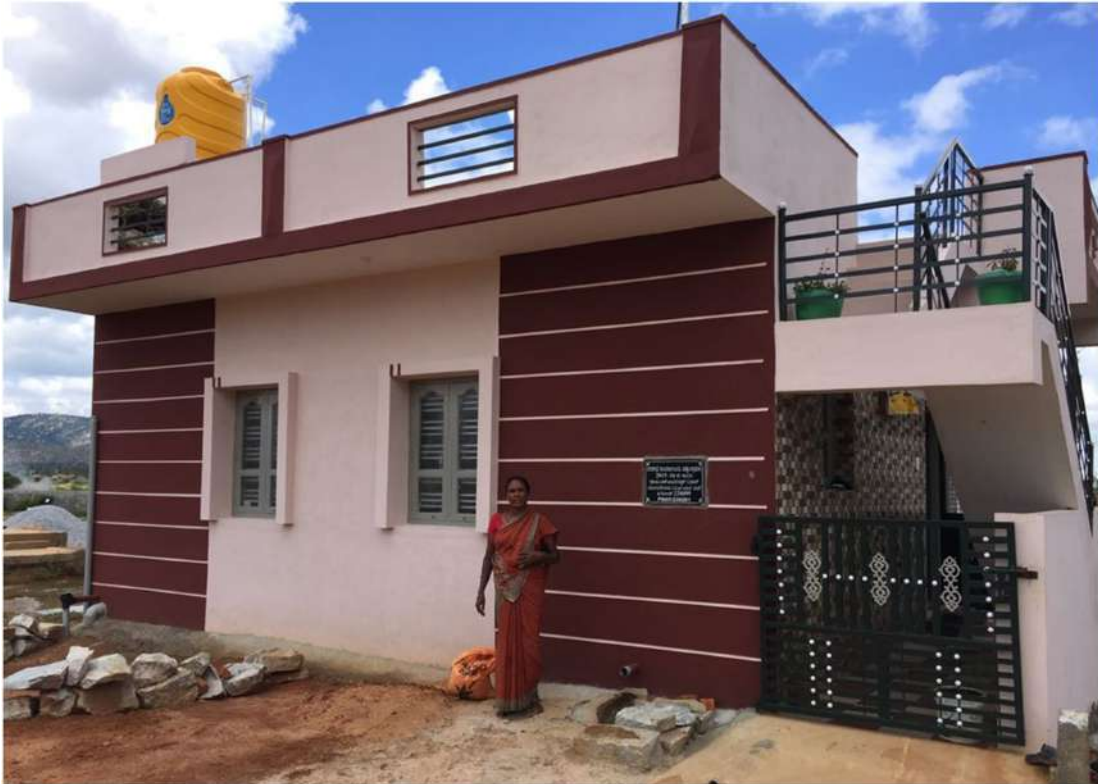
Beneficiary-Led Construction house under PMAY(U) in Chikkaballapur, Karnataka
