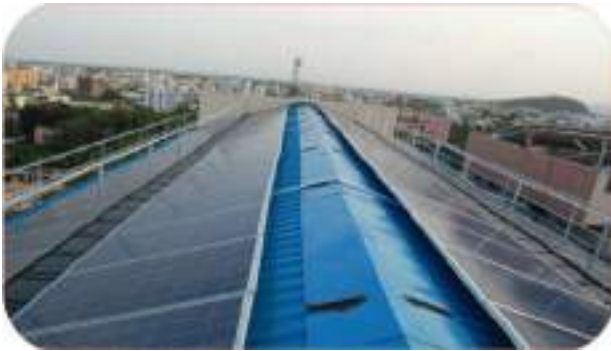
50 KWP roof top Solar Power Plant at CGO Complex, Vijayawada, Andhra Pradesh
