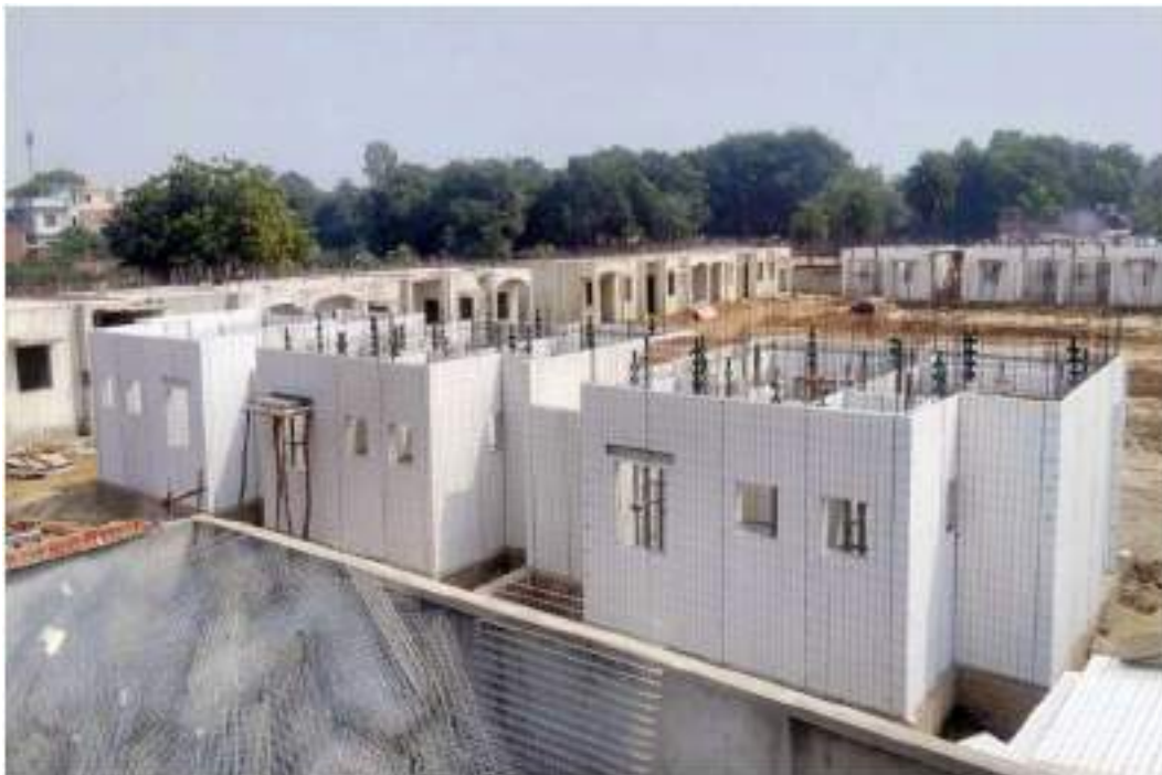
Demonstration Houses being constructed using Stay in Place EPS based double walled panel System by BMTPC at Aurangabad Jagir, Lucknow, Uttar Pradesh
