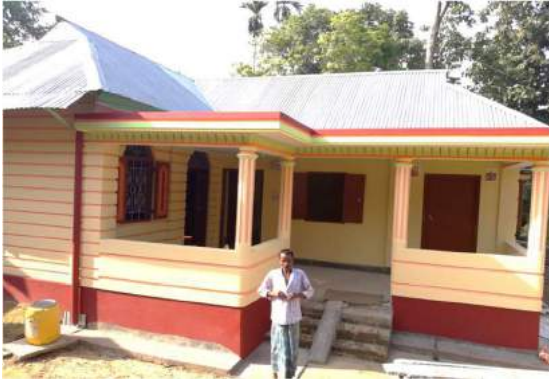
Beneficiary-Led Construction house under PMAY(U) in Amarpur, Tripura
