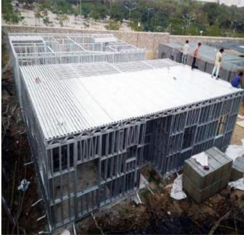
Demonstration Houses being constructed using Coffers Structural Stay in Place Formwork System (16 houses) and Light Gauge Steel Frame System (16 houses) by BMTPC at Gachibowli, Hyderabad, Telangana
