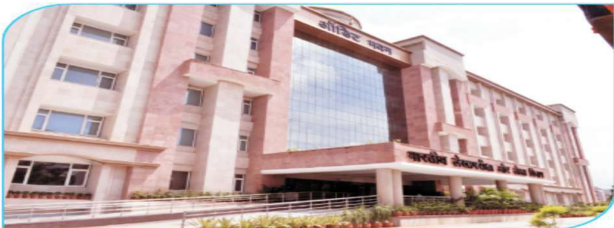
Audit Building, Lucknow
