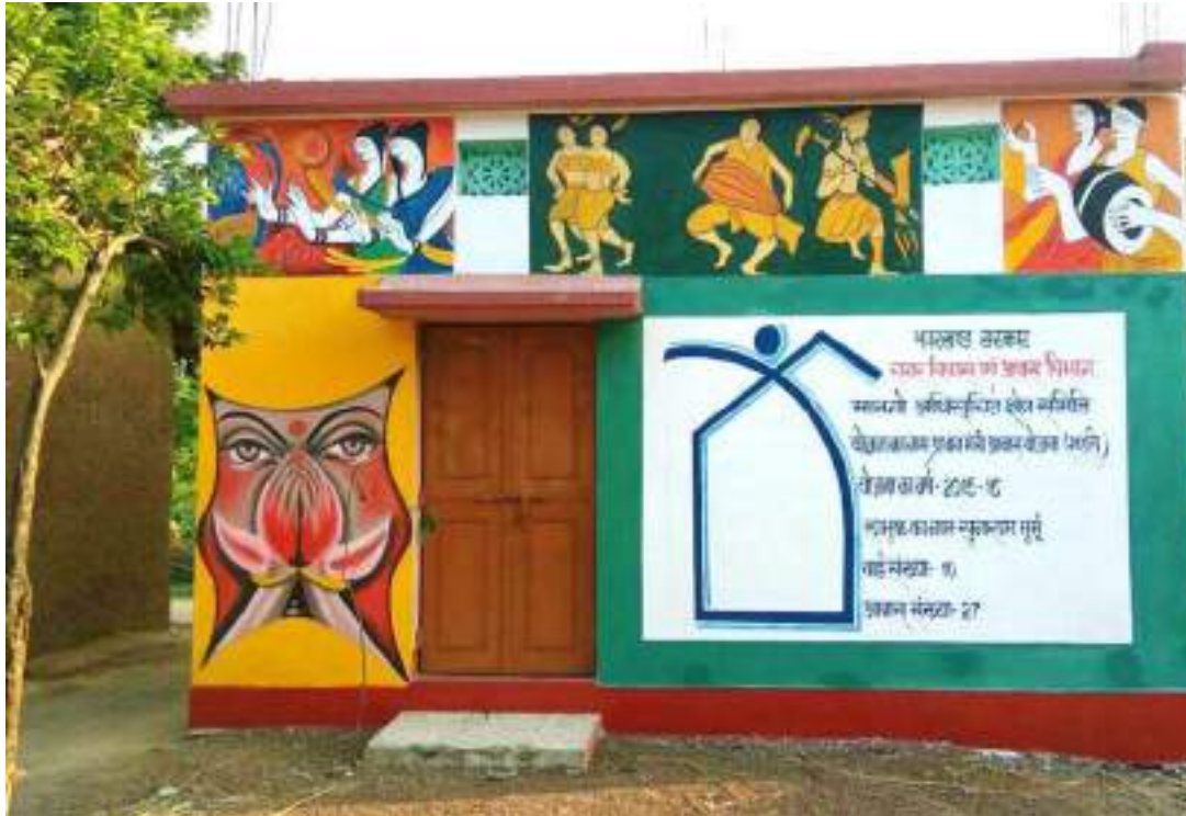
Beneficiary-Led Construction house under PMAY(U) in Maango, (Jamshedpur), Jharkhand
