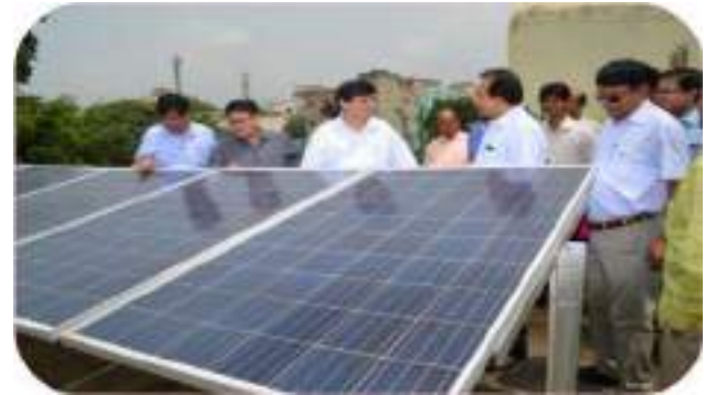
10 KWP roof top Solar Power Plant at CPWD Inspection Bungalow Ranchi Jharkhand
