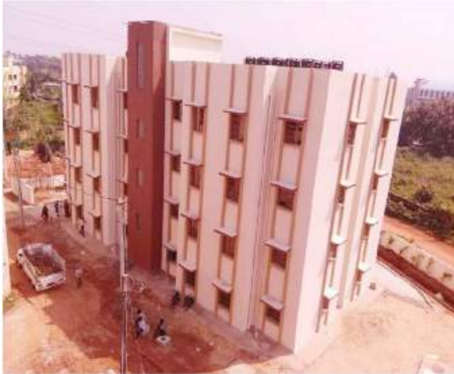
Demonstration Houses constructed using EPS technology by BMTPC at Bhubaneswar, Odisha
