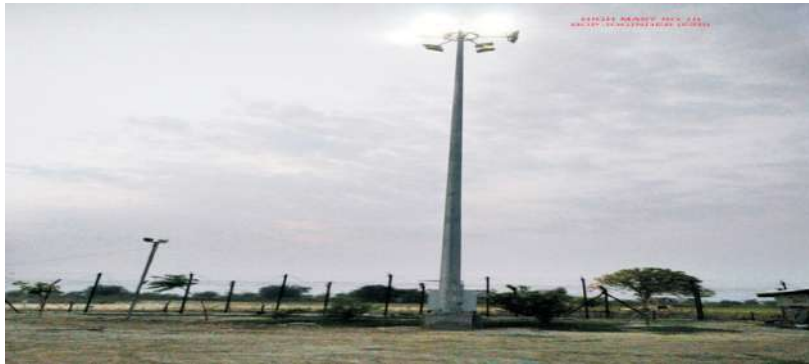
High Mast BOP Joginder, Firozpur, Punjab
