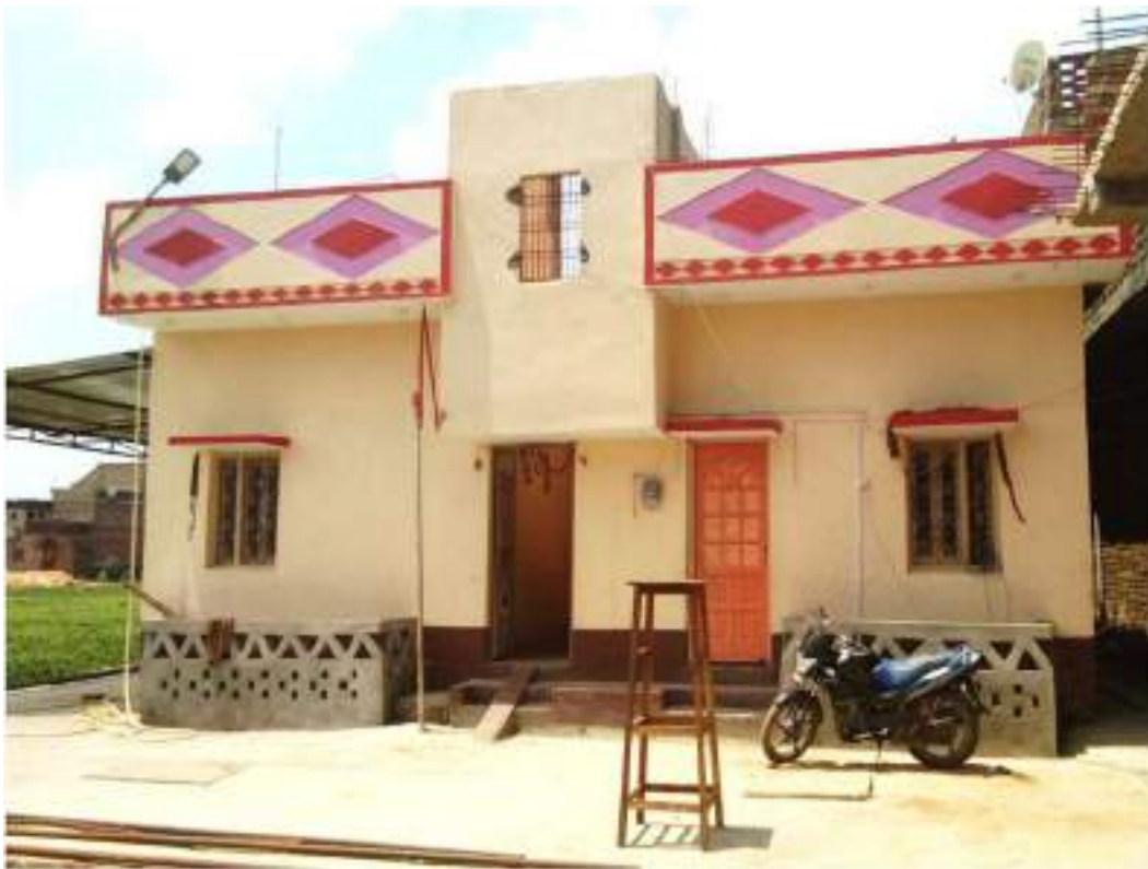
Beneficiary-Led Construction house under PMAY(U) in Gaya, Bihar
