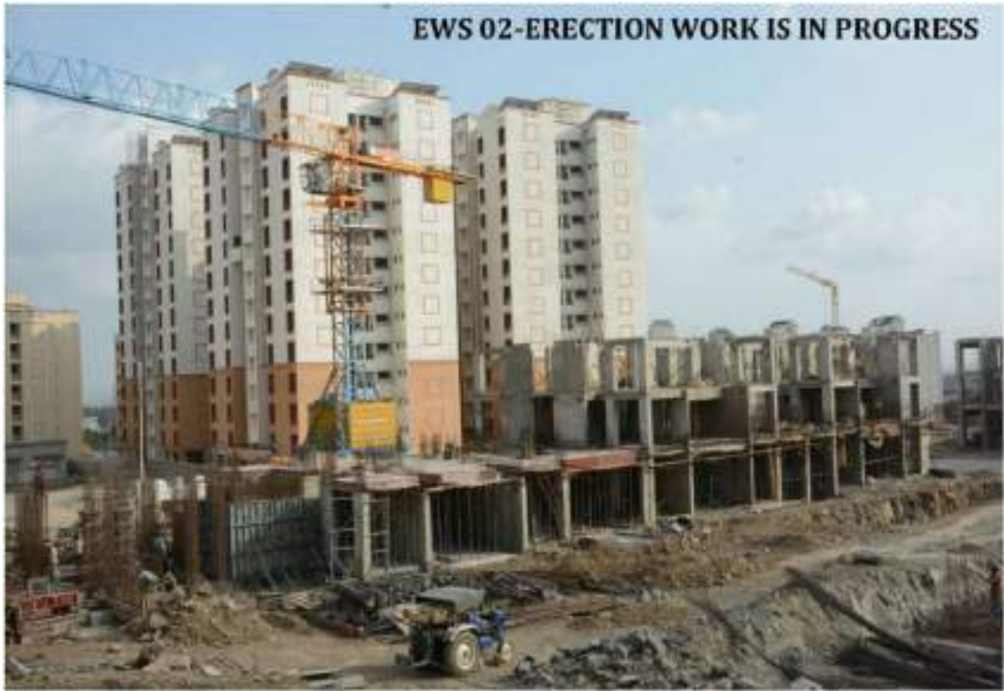
AHP houses in Pune, Maharashtra using Precast Construction Technology
