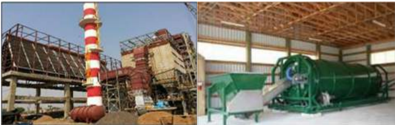
Waste to energy plants
