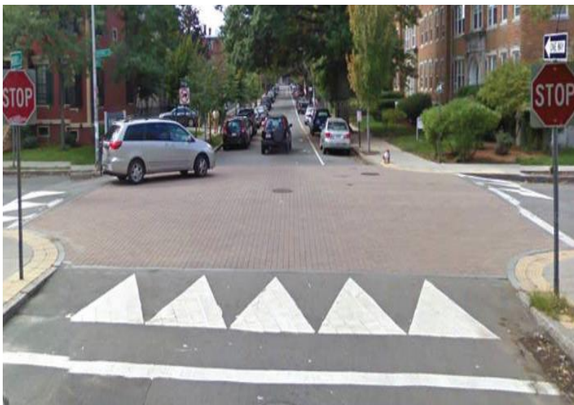
Figure 6-20 : Concept layout of non-signalised 4-arm junction with raised pedestrian crossing
