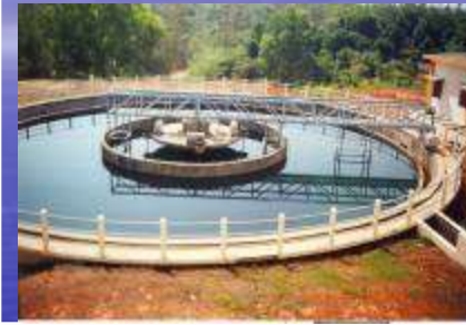
WTP Clarifier and Lab Facilities
