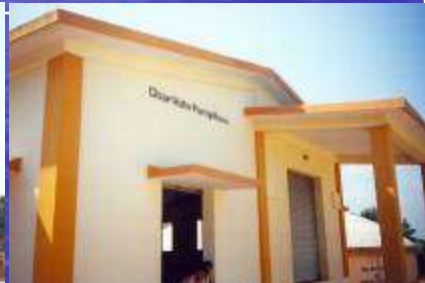
WTP Chemical house and Clear Water Pump House
